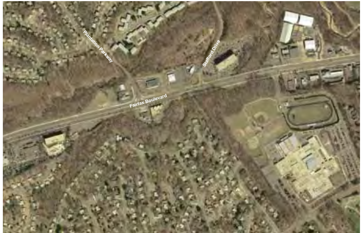
Aerial view of the East Connector
