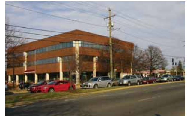
Existing office building
