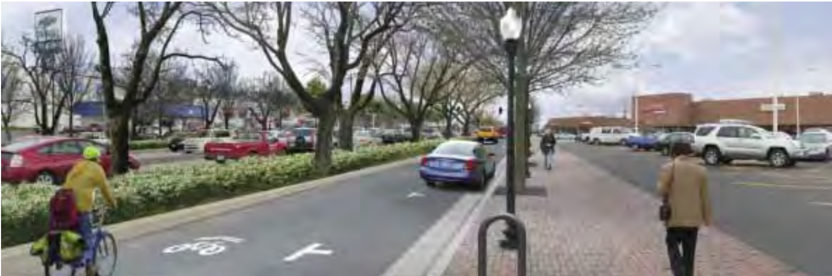
Initial Improvements: A slow lane is added parallel to the Boulevard, forming the framework for a proper grand boulevard. A second row of street trees are planted and a wide sidewalk is included adjacent to the slow lane. On-street, parallel parking is included within the slow lane, providing the foundation for street-oriented buildings. The slow lane includes a narrow travel lane which decreases the speed of vehicles, making the street a safe and comfortable place for cyclists, pedestrians, and vehicles.
