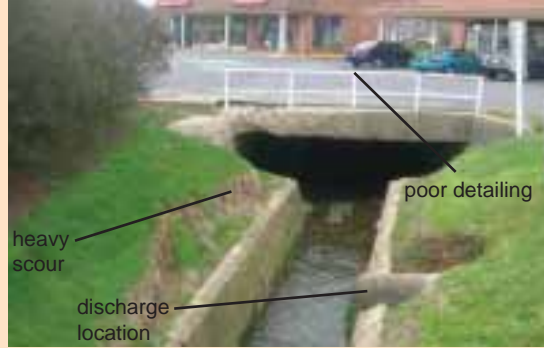
North Fork Accotink Creek heads underground when it reaches Fairfax Shopping Center.
