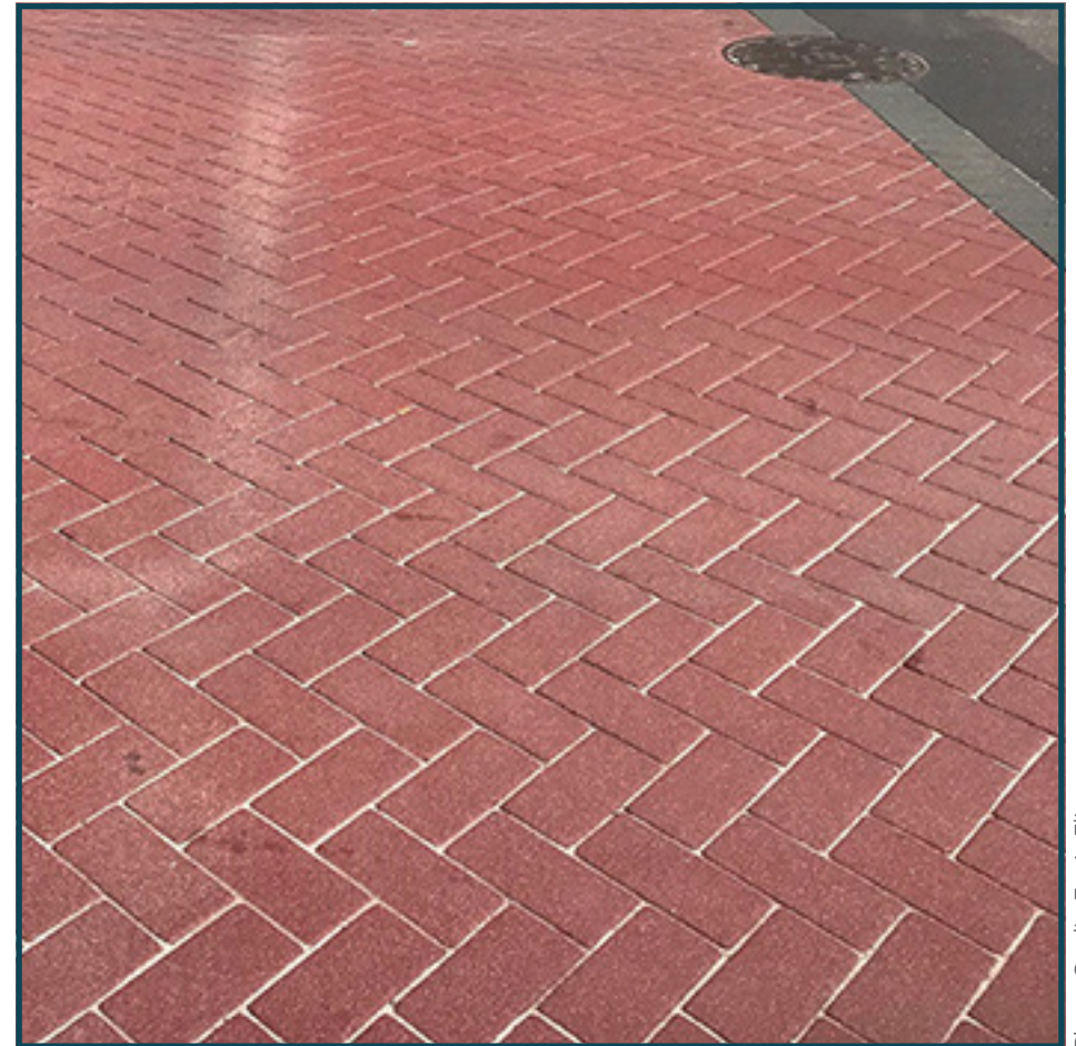
TrafficPatternsXD® installed on Broad Street, Philadelphia, diagonal herringbone pattern
