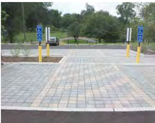
Figure 49. Example of permeable pavers in a parking lot at Riverside Park in Lynchburg, Virginia.
