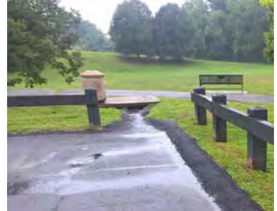
Figure 23. Surface drain from the parking lot to an inlet drain
