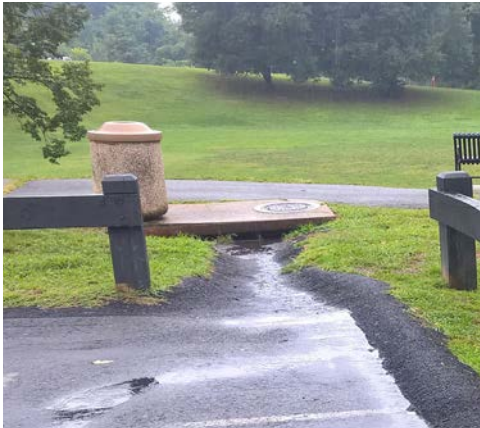
Figure 18. Surface runoff from existing parking lot
