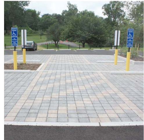
Figure 53. Example of permeable/pervious pavers in a parking lot
