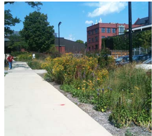
Figure 54. Bioretention or rain garden plantings adjacent to a parking lot
