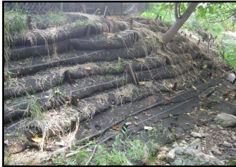
Figure 6: Filtrexx Socks at Daniels Run
