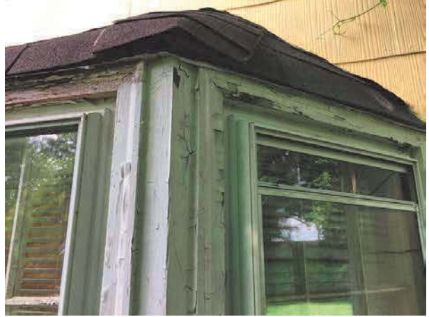
Shingles over bay window
