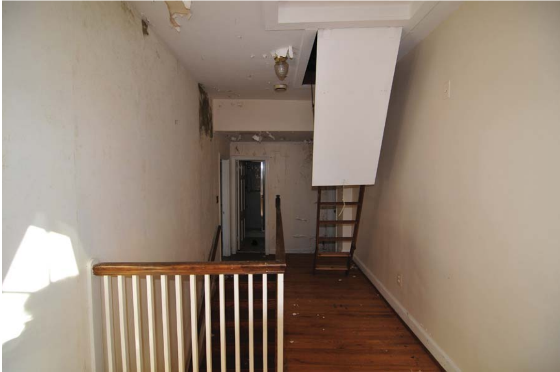
1911 Floor 2 Hallway View N.JPG
