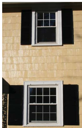
View of non-original windows in the original portion of the building
