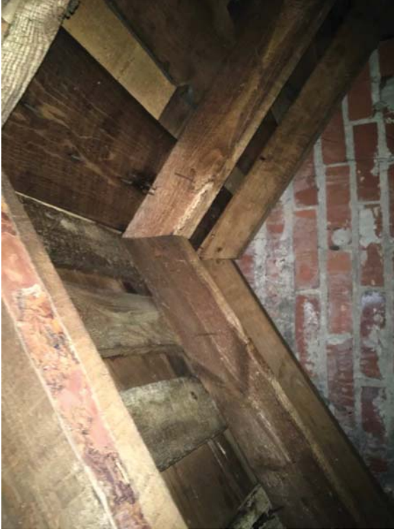
Typical main building gable roof framing.
