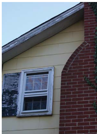
View of storm window on 1970 addition, 2nd floor, north facade
