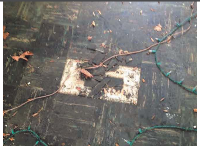
2. View of the 9" x 9" black floor tiles (ACM), Samples 1-2.
