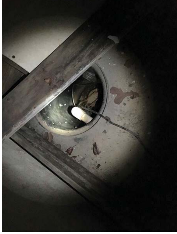
Sump pit within Cellar level. Pit was dry.
