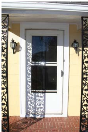
View of front door screen
