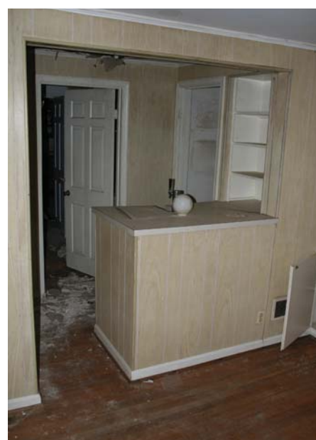
View of family room bar looking northwest
