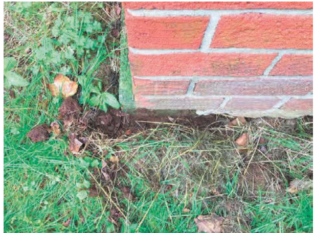
Rear chimney bottom
