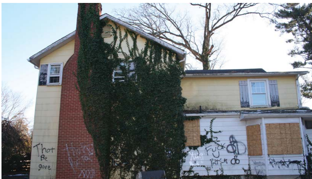
View of North facade looking South
