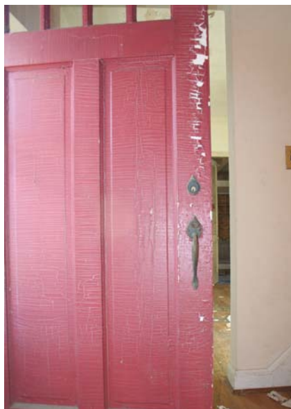
View of front door
