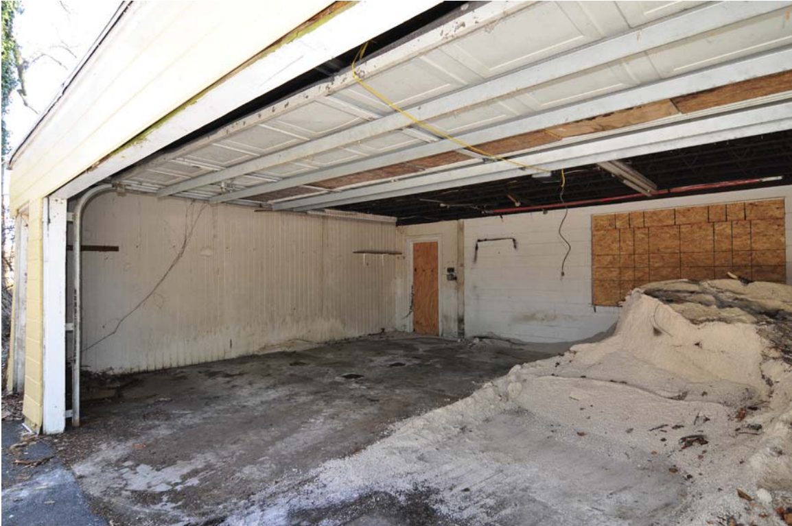
1955 Floor 1 Attached Garage View NE.JPG
