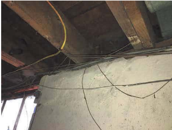
Organic growth penetrating from outside into basement
