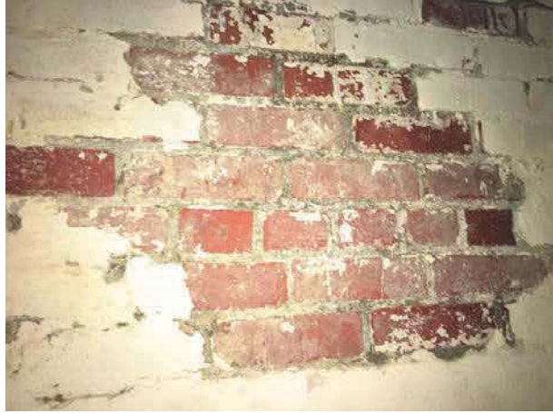
Exposed area of basement wall
