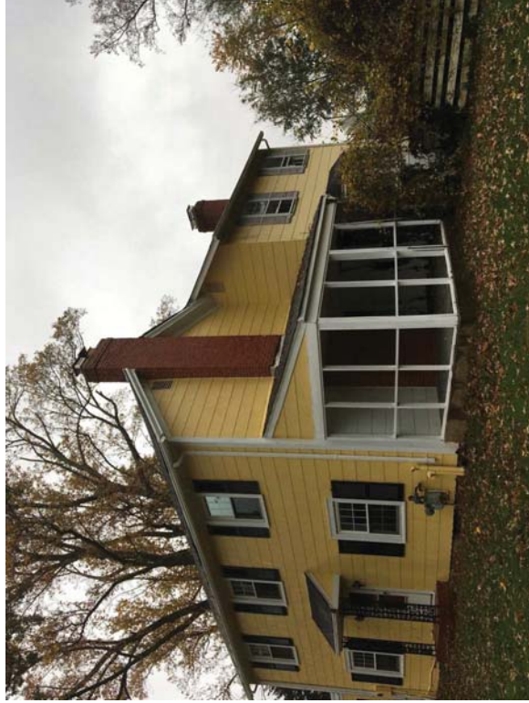
Southeast corner of building.
