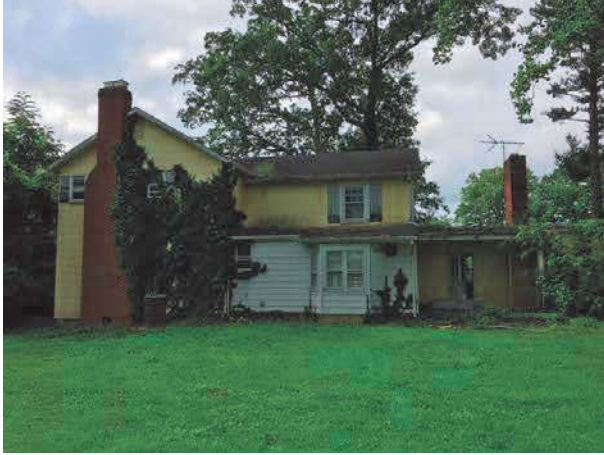
Flat roof at garage and laundry area
