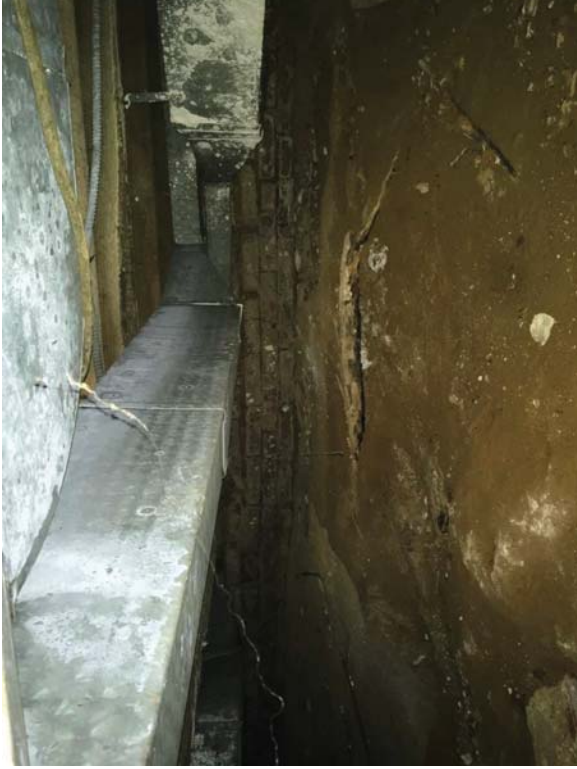
Crawl space under main portion of structure.
