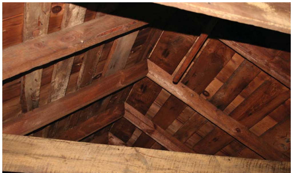
View of roof framing in original portion of the house
