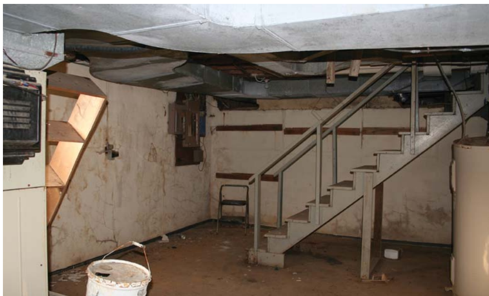
View of basement looking southwest
