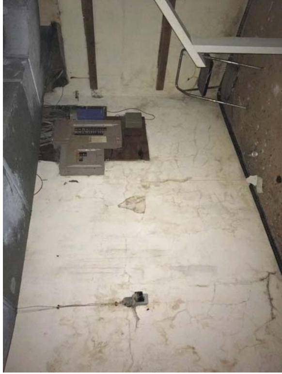
Cellar level under structure.
