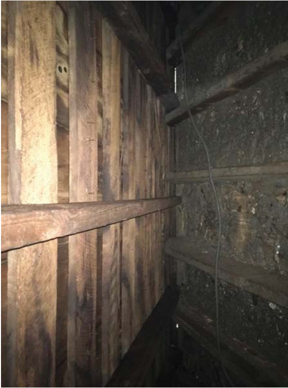
Typical roof rafter.
