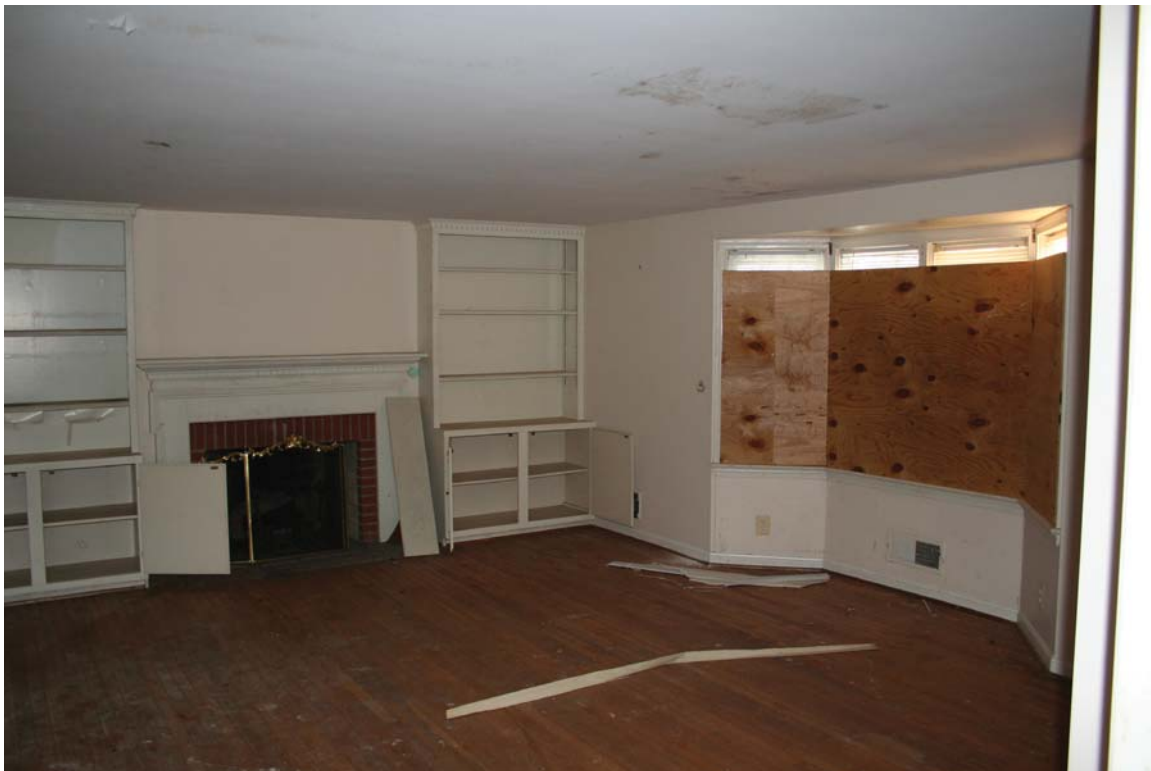
View of Family Room looking northeast
