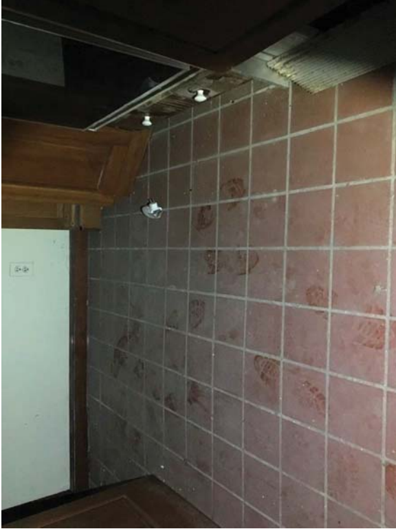
Significant displacement of floor structure within kitchen. Estimated 1.5" within five feet.
