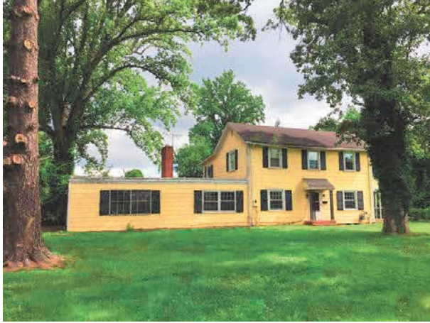
Gutters at the front
