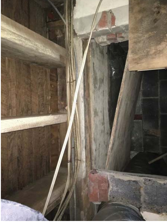
Floor support beam spanning opening.
