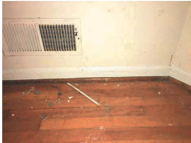
Dry wall with hardwood floor
