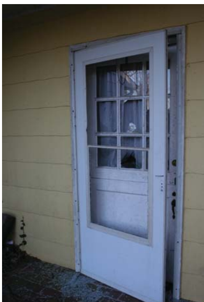
View of exterior door into Den
