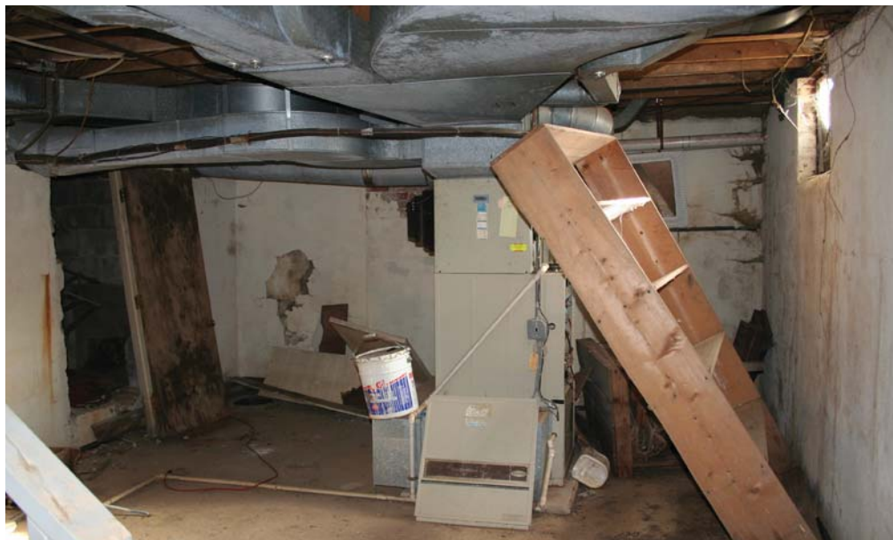
View of basement looking Northeast, note wood framing under 1st floor
