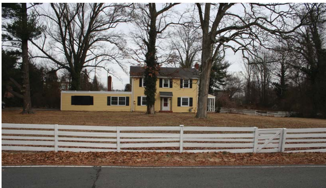
View of South Facade
