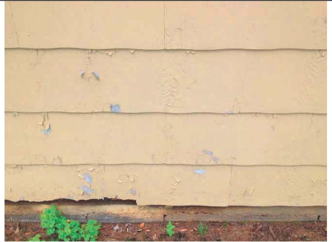
22. View of the cement board siding (ACM), Samples 73-74, and paint chips in the drip line.
