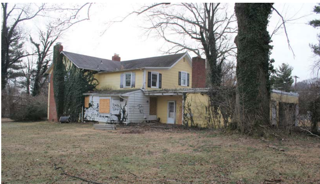
View of North Facade, looking Southeast
