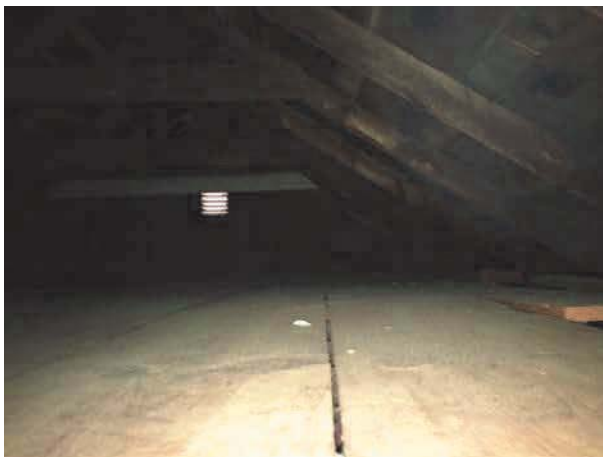
Rafter system supporting roof
