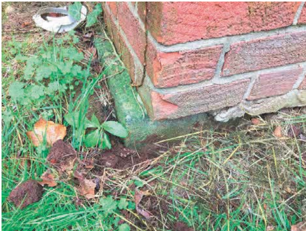
Rear chimney bottom
