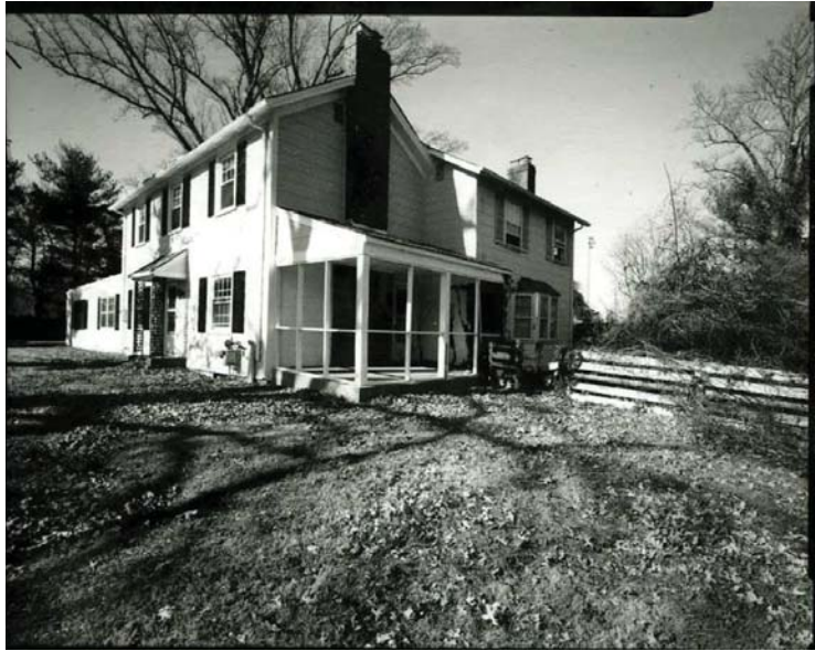
Facade, Screen Porch, 1972 Addition View NW.JPG
