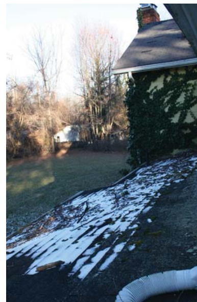
View of roof over kitchen
