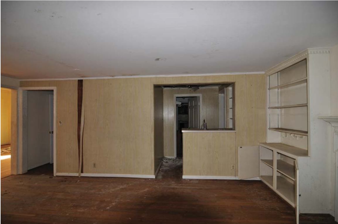
1972 Floor 1 Family Room View W.JPG
