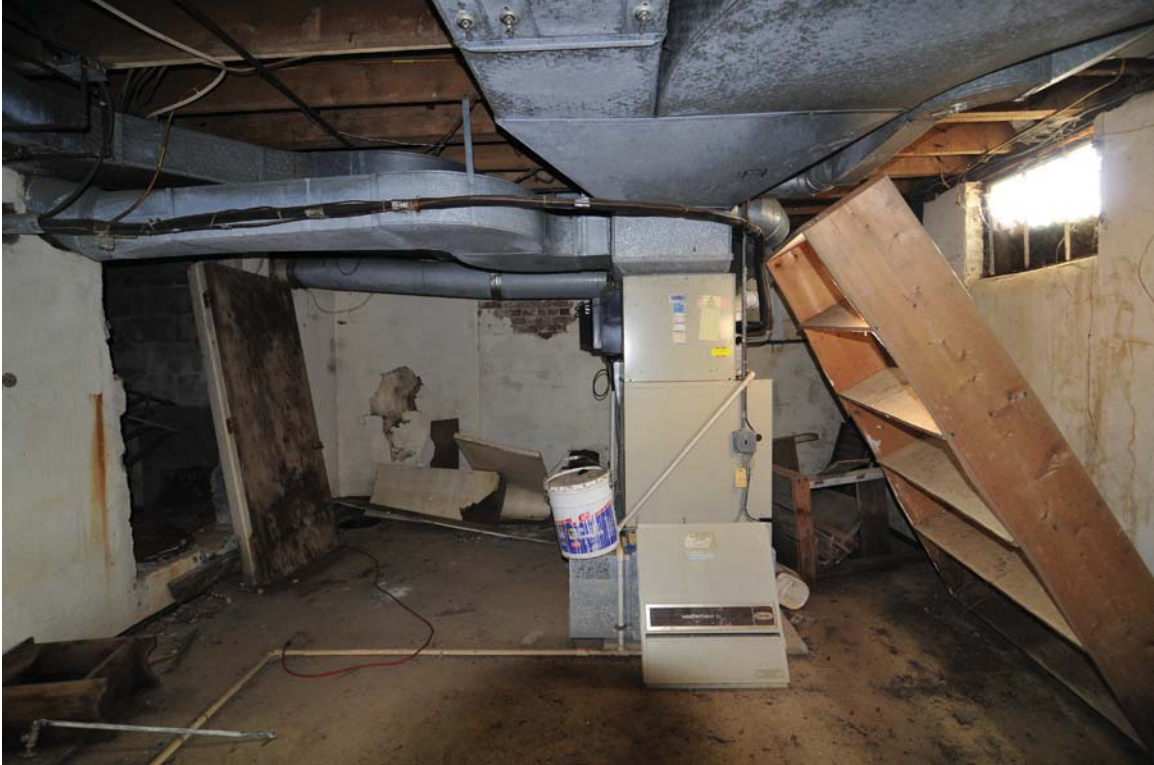
Basement View E.JPG
