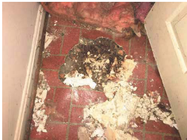
Flooring in the laundry room
