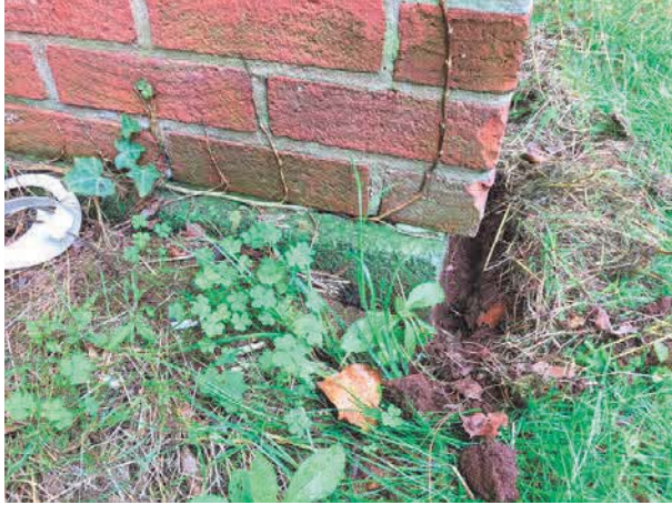
Rear chimney bottom
