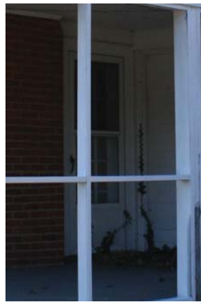
View of screen door of exterior door from Porch into Living Room
