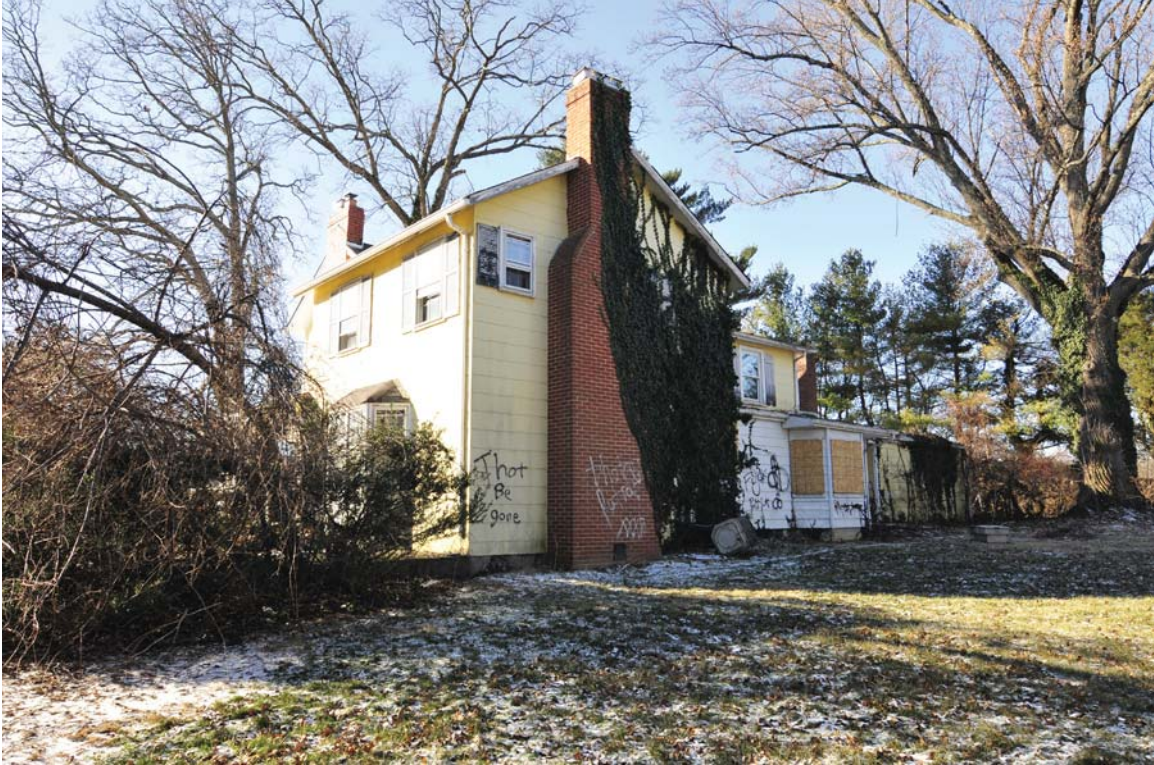
1972 Rear Wing Addition View SW.JPG
