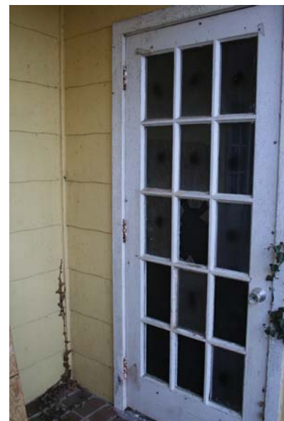
View of door into garage from Patio 2
