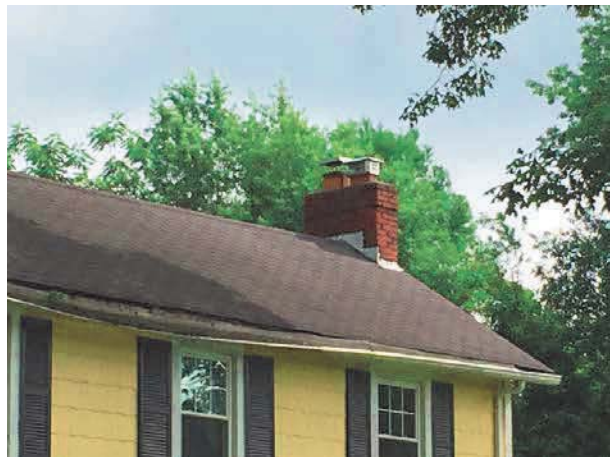
Typical roof condition
