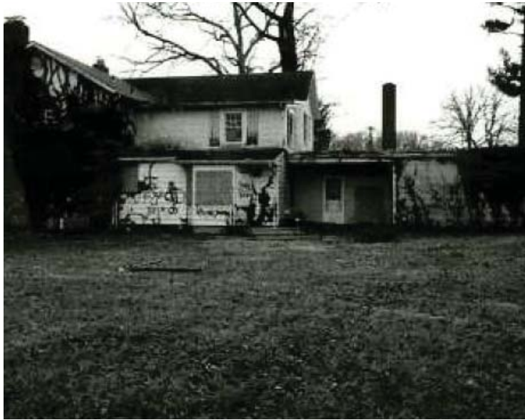
Rear Elevation View South.JPG
