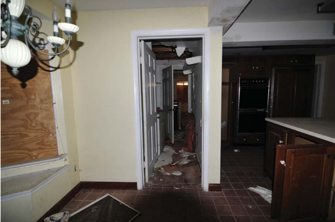
1972 Floor 1 Kitchen and Hall View E.JPG
