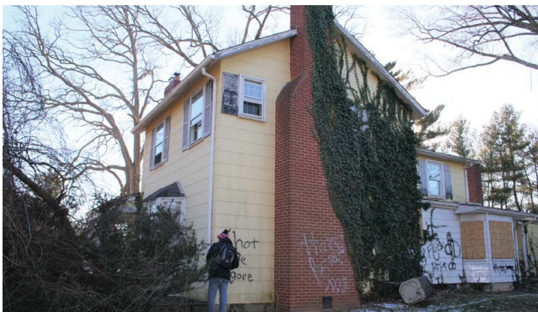
View of north chimney
