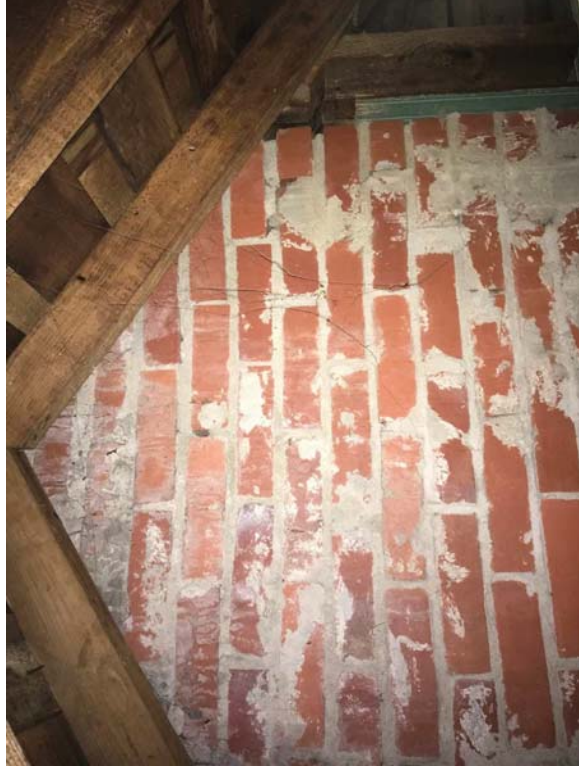
Brick wall at gable end.
