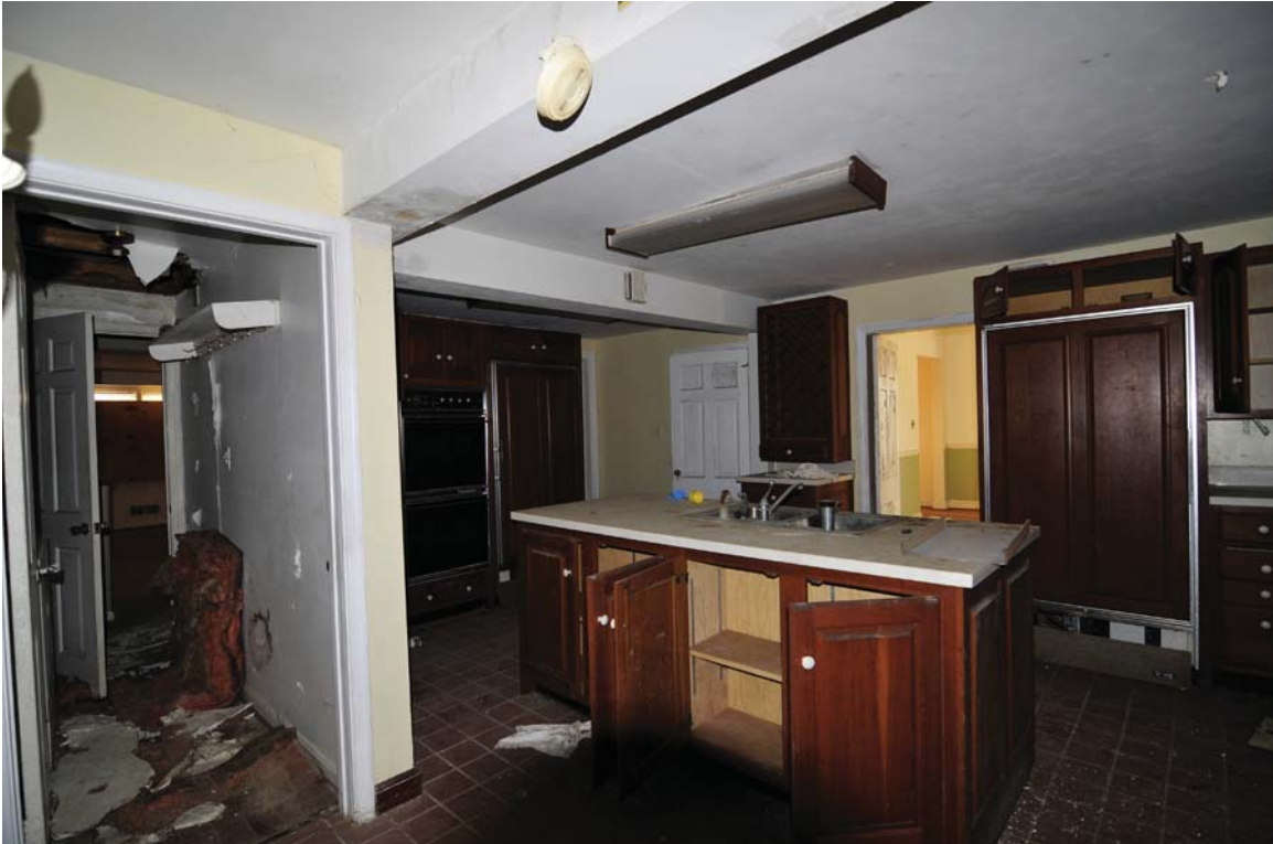
1972 Floor 1 Kitchen View SW.JPG
