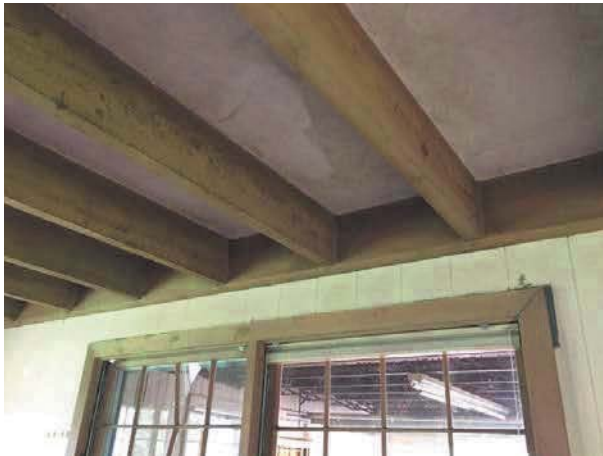
Exposed joists in room adjacent to garage
