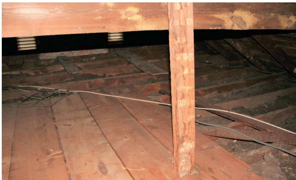
View of Insulation in attic, above original footprint of the house
