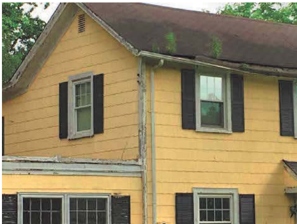
Typical roof condition
