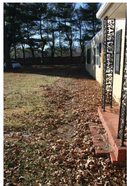
View of front walkway
