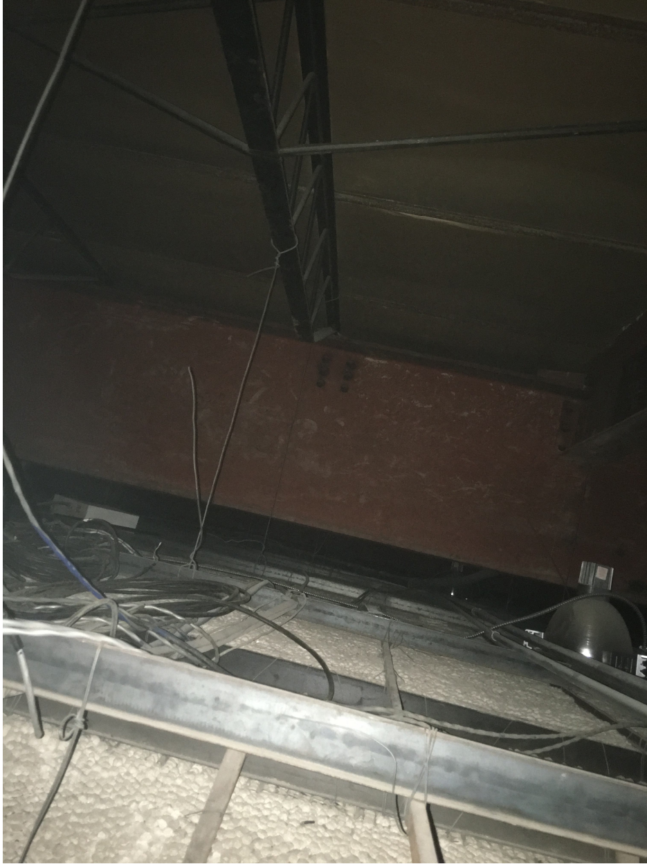
Photo #4: Steel beam supporting roof joists at corridor bearing line
