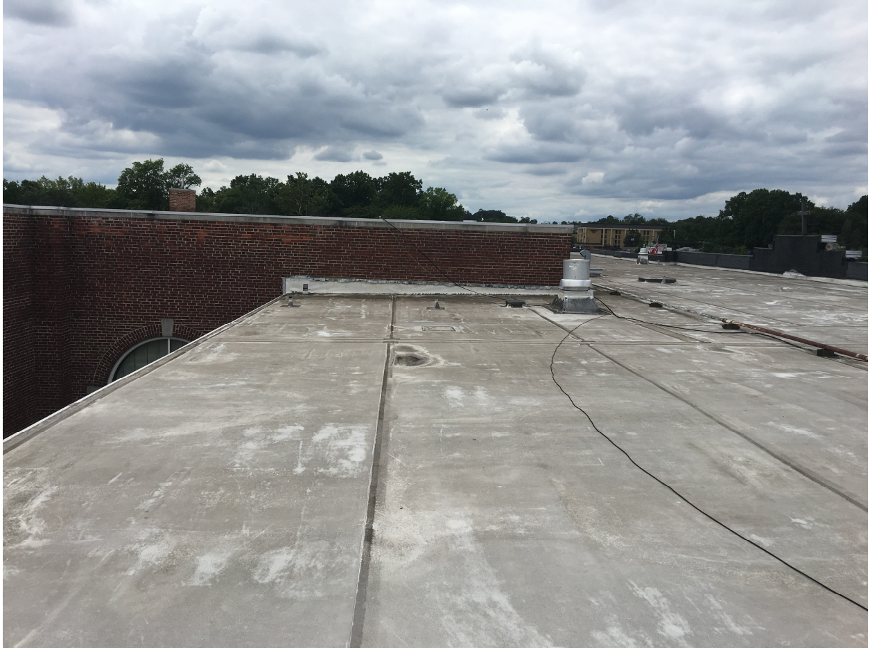
Photo #5: Parapet walls pop-up at Library and Cafeteria wings
