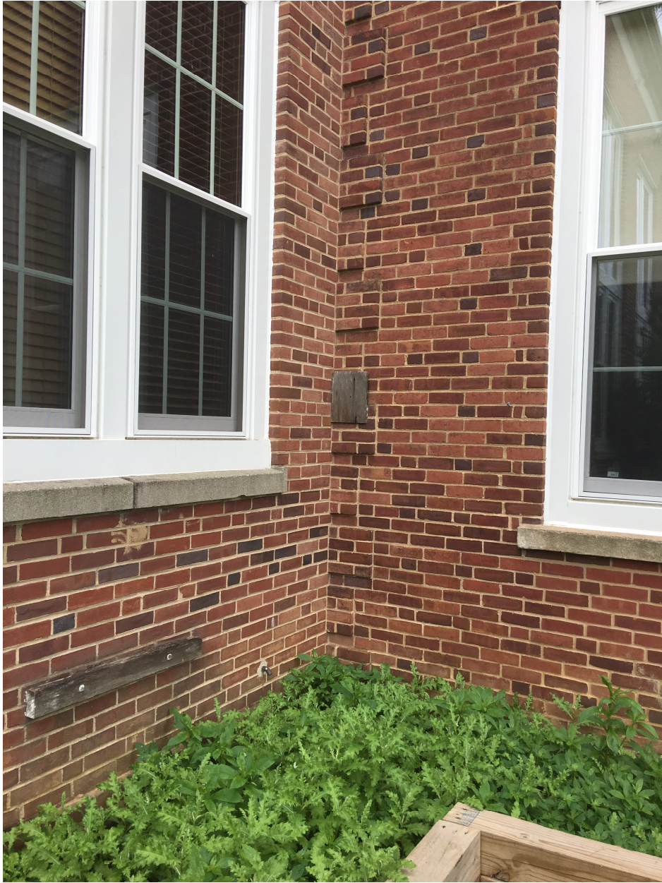
Photo #6: Front elevation at building corner
