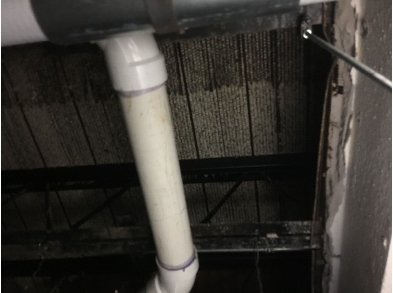
Photo #1: Underside of 2 nd floor joists with metal lath decking
