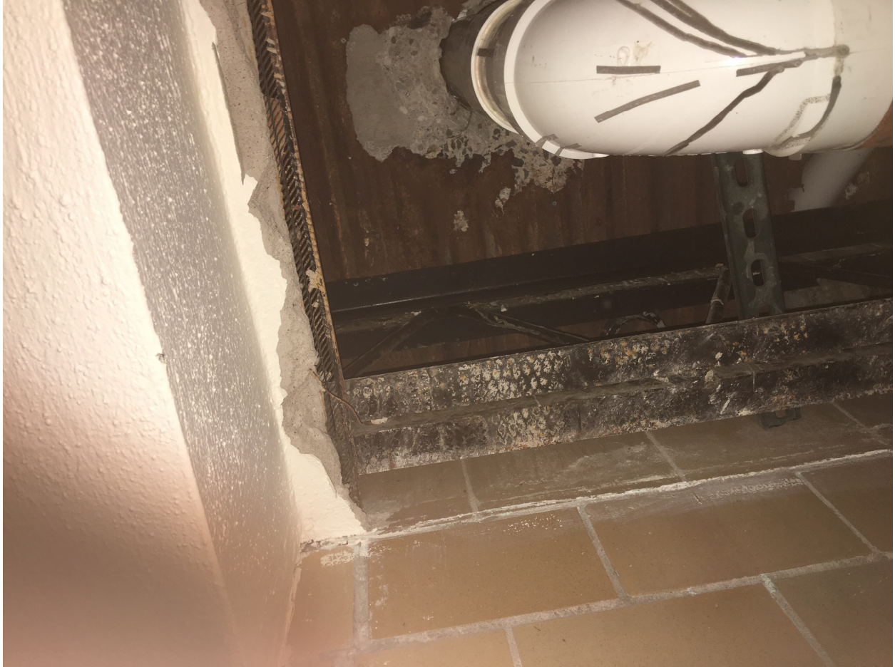
Photo #2: Underside of 2 nd floor joists with steel form decking
