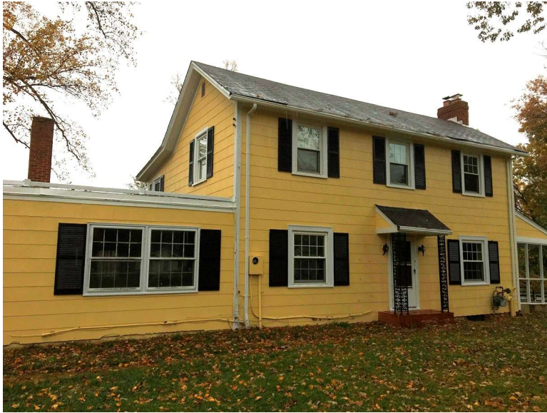
Front elevation / main entrance of property. South facing.
