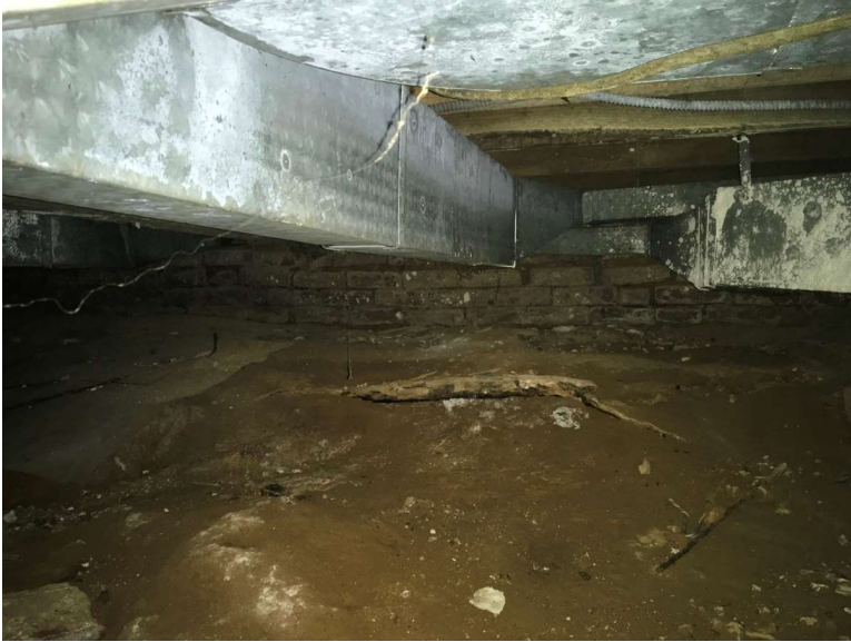
Crawl space under main portion of structure.
