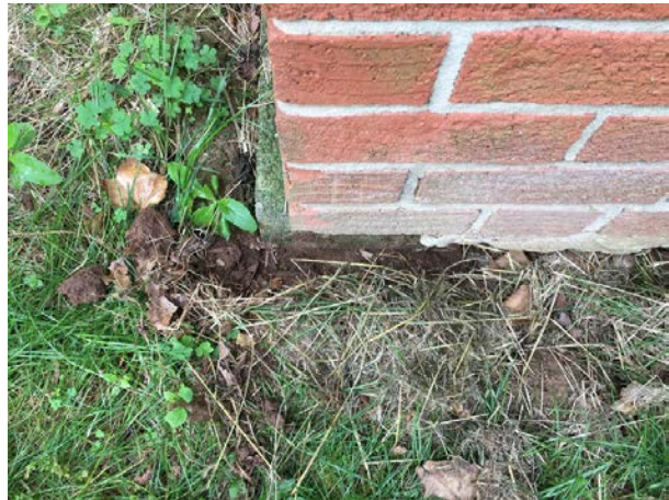
Rear chimney bottom
