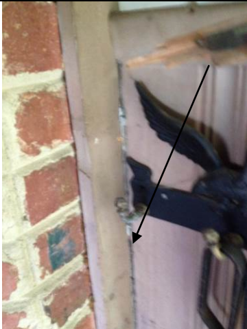
3. View of the light gray wall caulk, Samples 5-6.
