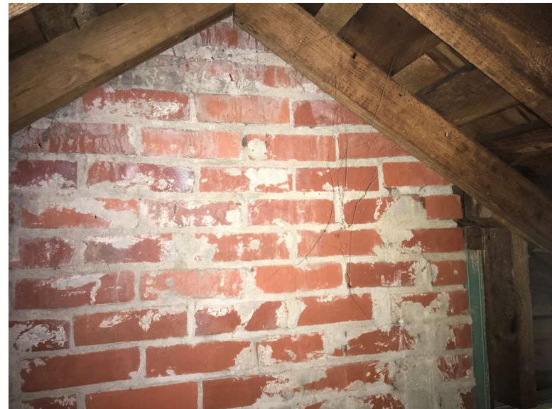
Brick wall at gable end.
