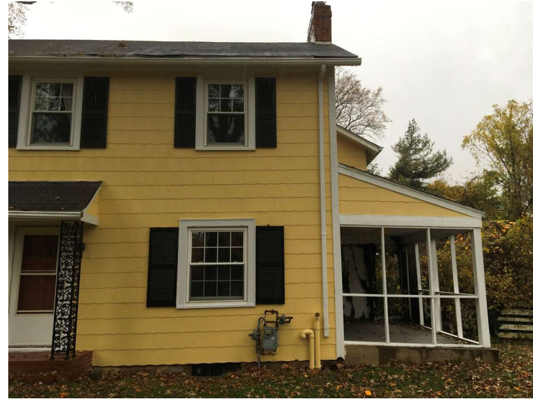
South elevation of property.
