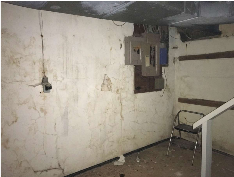
Cellar level under structure.
