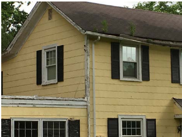
Typical roof condition
