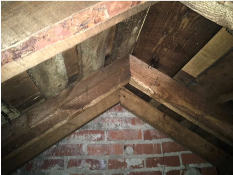
Typical main building gable roof framing.
