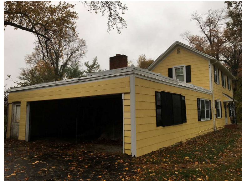
West side of building.
