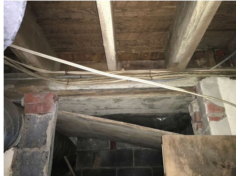
Floor support beam spanning opening.
