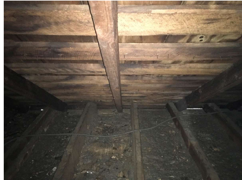
Typical roof rafter.
