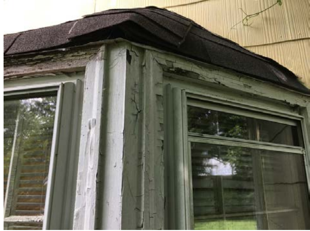
Shingles over bay window
