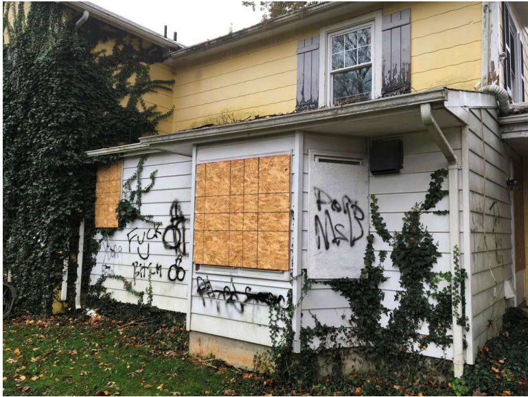
North elevation of property.
