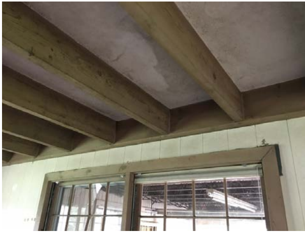
Exposed joists in room adjacent to garage
