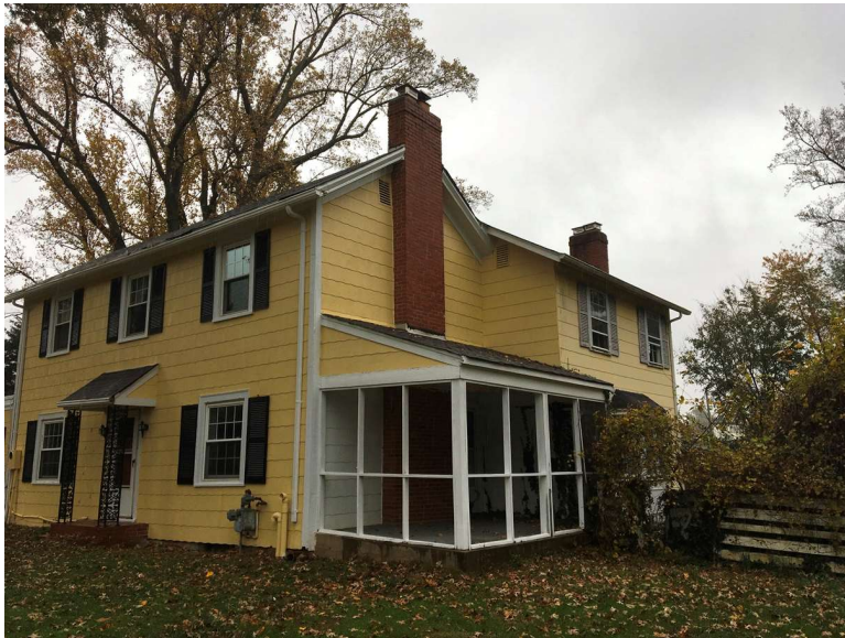
Southeast corner of building.
