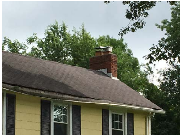
Typical roof condition
