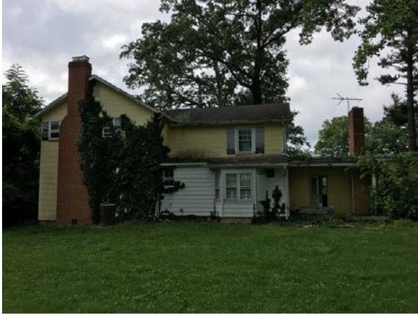
Flat roof at garage and laundry area
