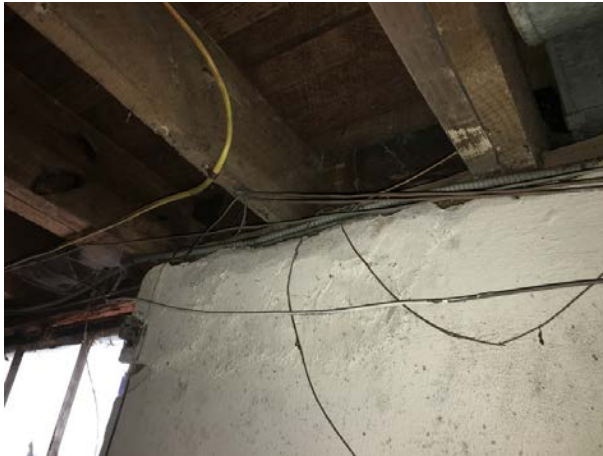
Organic growth penetrating from outside into basement
