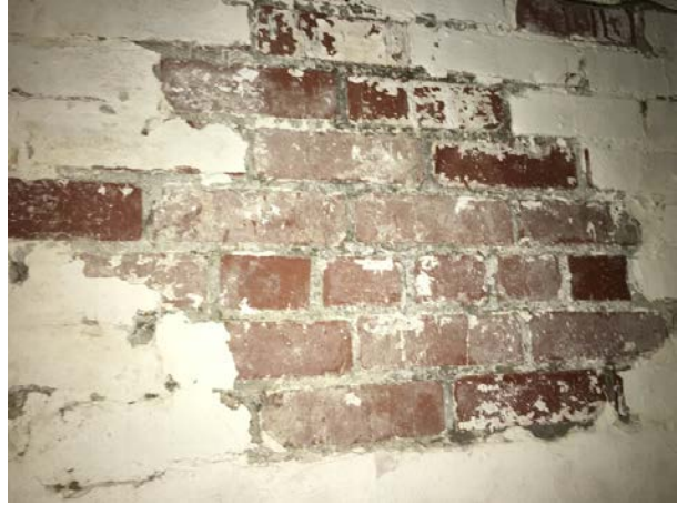
Exposed area of basement wall
