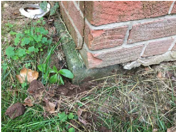
Rear chimney bottom
