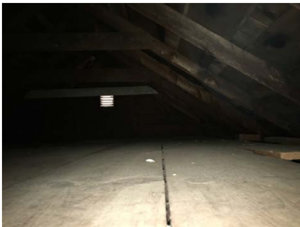
Rafter system supporting roof
