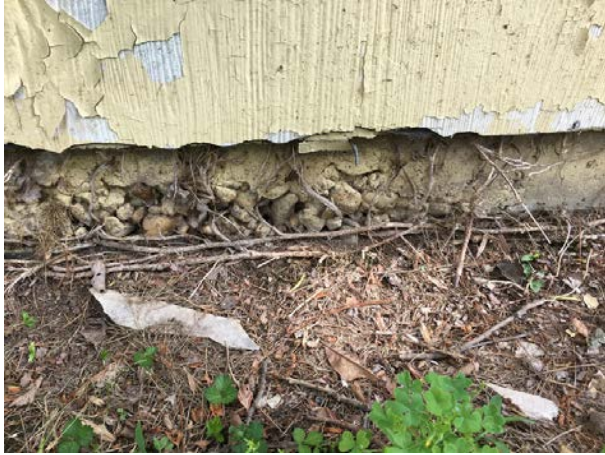
Organic grow into the wall
