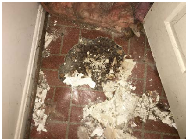
Flooring in the laundry room
