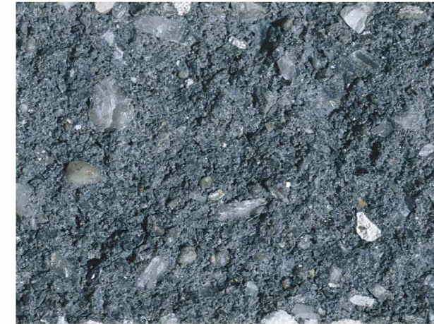
CMU-1 Concrete Masonry Unit, Exterior Perimeter of Building
