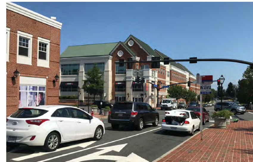
No pedestrian amenities or buffer from vehicular traffic along North Street
