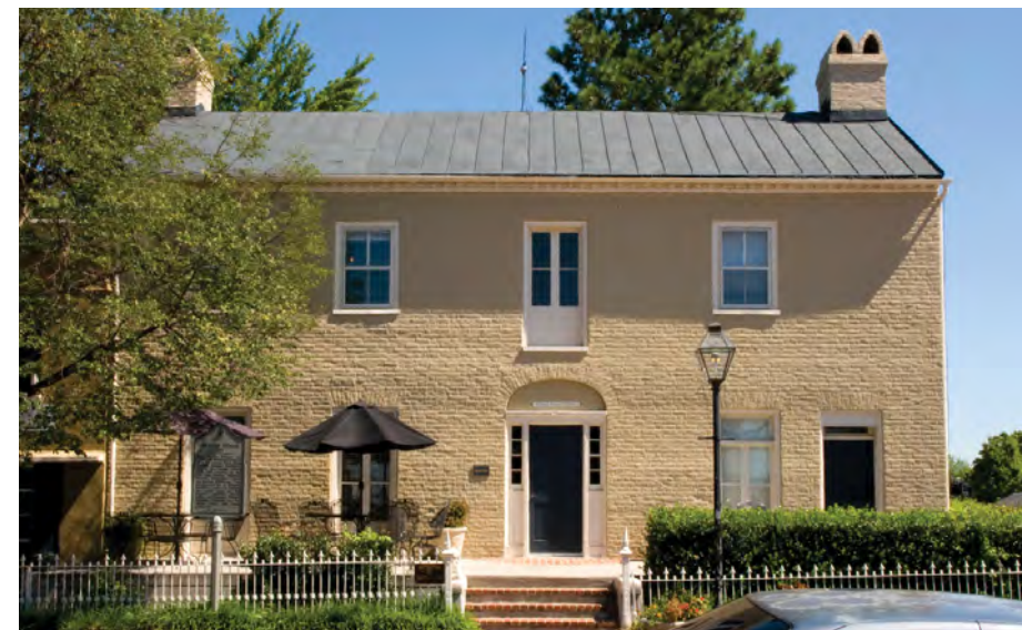
Draper Building, Main Street Old Town, Fairfax City
