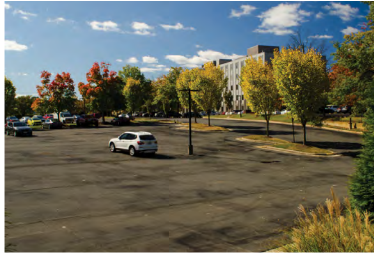
WillowWood Plaza Parking Lot Looking South
