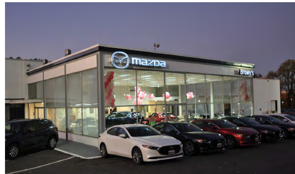
Above - Existing Photo of Browns Mazda
