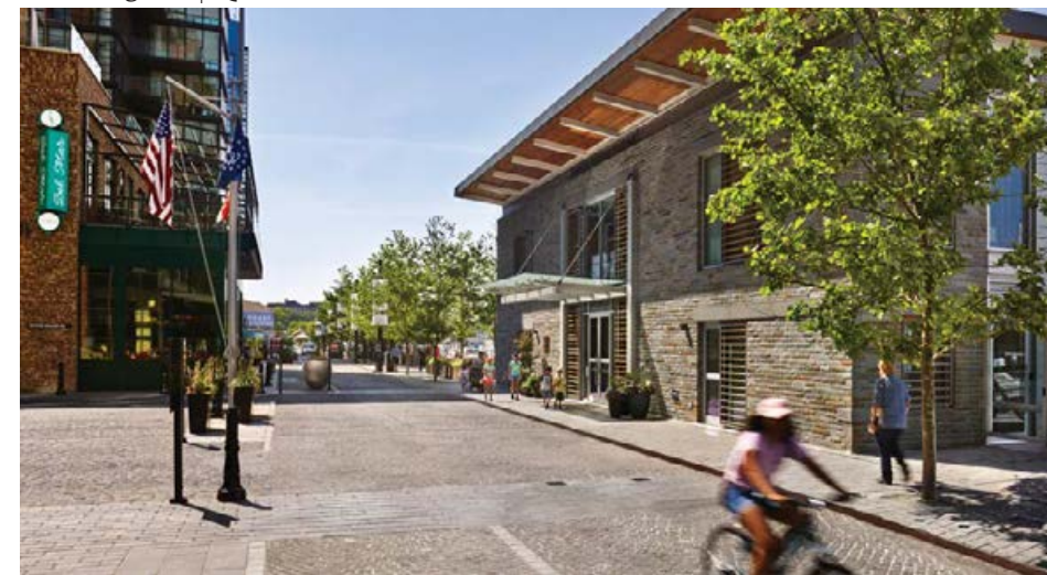
The Wharf's Capital Yacht Club in Washington, DC designed by Cunningham Quill Architects fronts a walkable pedestrian oriented street.
