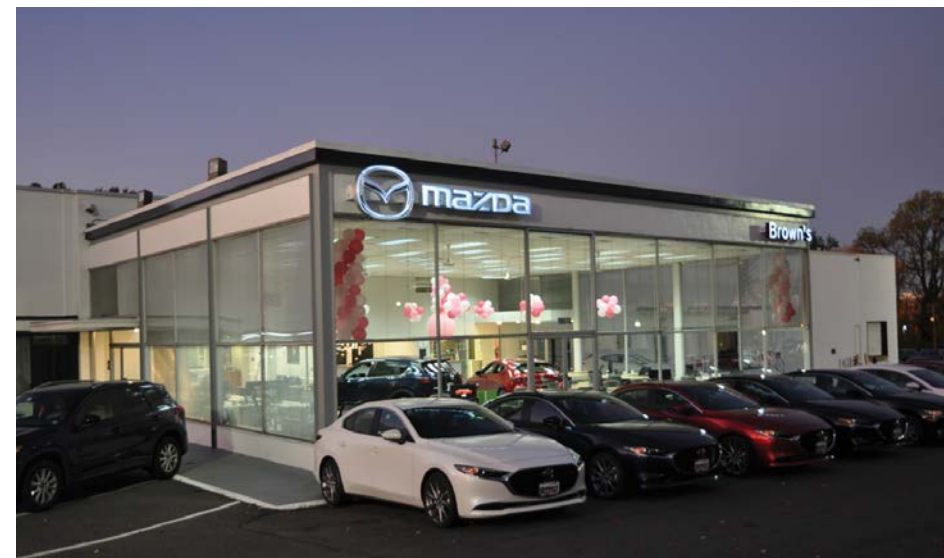
Above - Existing Photo of Browns Mazda
