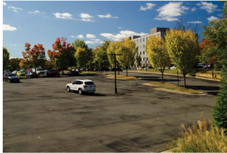
WillowWood Plaza Parking Lot Looking South
