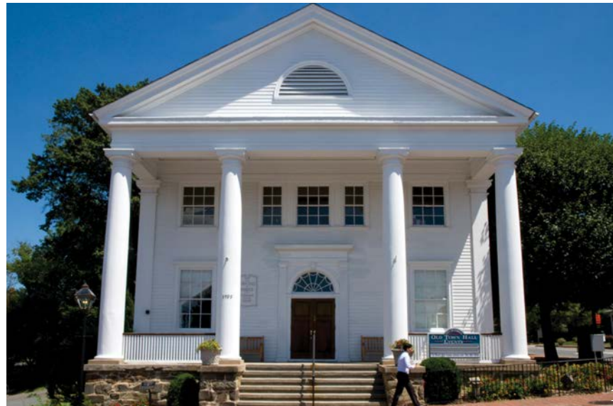
IMAGES: 1. Old Town Hall in Old Town 2. 29 Diner in Northfax 3. View of North Street- part of the transition overlay district of Old Town.
