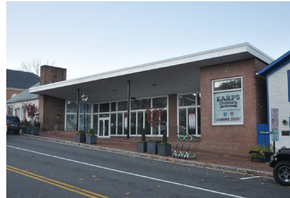
Building along 10426 Main Street
