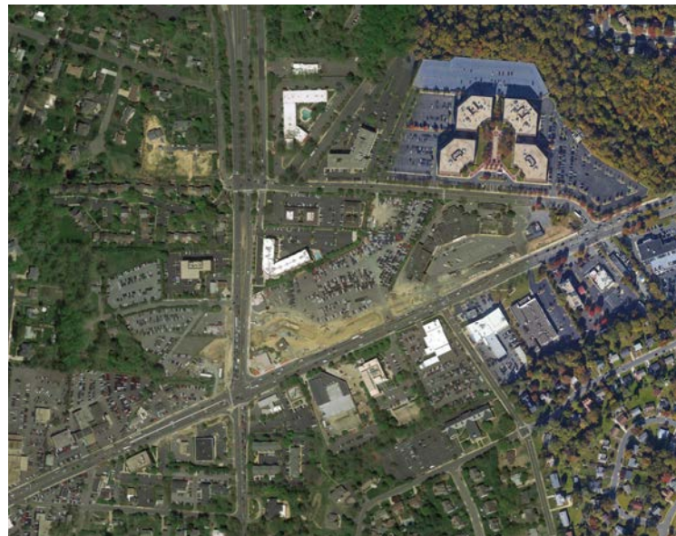
Land Use Dominated by Parking & Impervious Surfaces in Northfax 20
