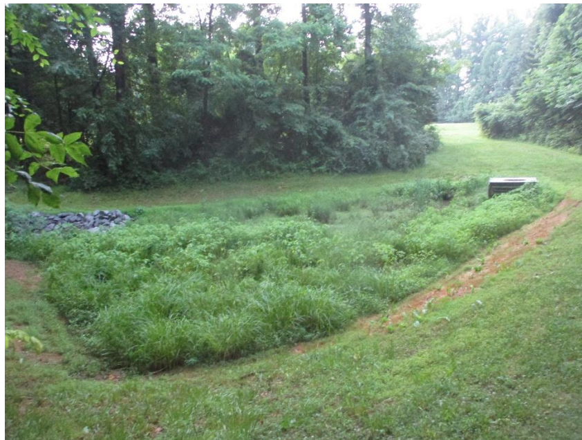
Figure 4. On-site detention pond (Fairfax BMP #2010010210) cleared of sediment and debris (2020)
