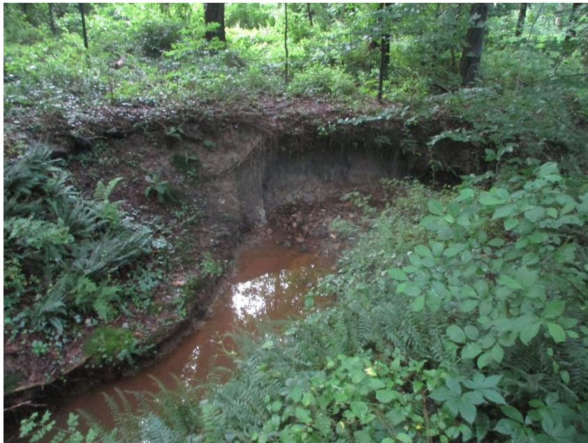
Figure 8. High bank erosion in the Popes Head Creek stream system
