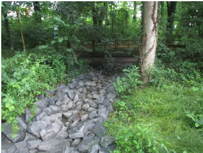
Figure 6. Stabilized, stone-lined inflow channel (2020)
