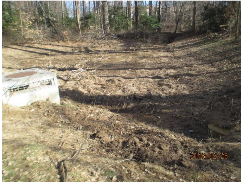
Figure 3. On-site detention pond (Fairfax BMP #2010010210) with enhanced sedimentation (2016)
