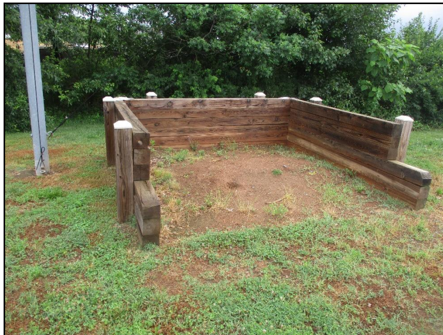
Figure 5. On-site field maintenance aggregate storage.
