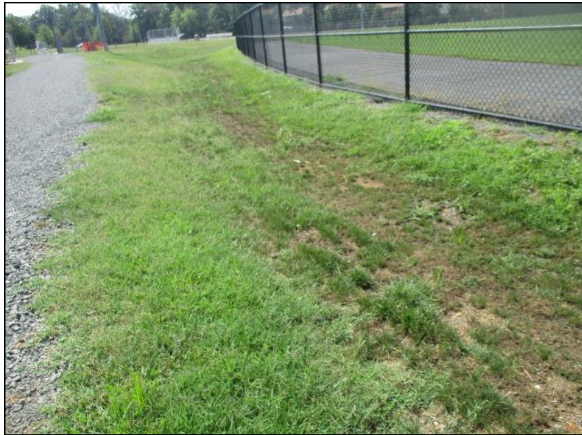
Figure 7. On-site Vegetated Swale with enhanced sediment loading and denuded channel banks (2016).
