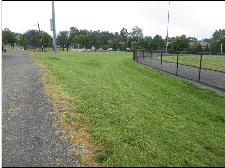
Figure 8. On-site Vegetated Swale with reduced denuded area (2020).
