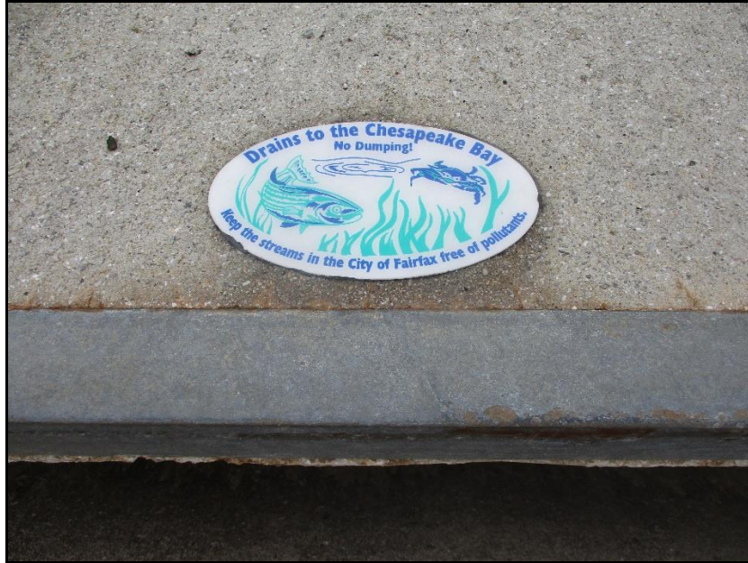
Figure 12. Storm Drain Marker (Typical).
