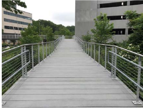
Deck: Concrete planks, 14-ft clear width (left), savannah brown color (top right), wood texture (bottom right)
