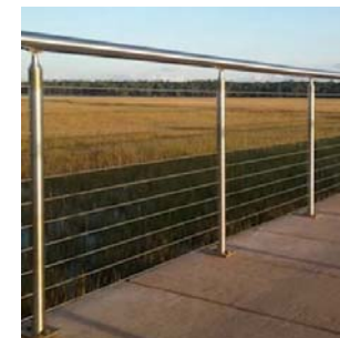
Stainless Steel with tensioned cable
