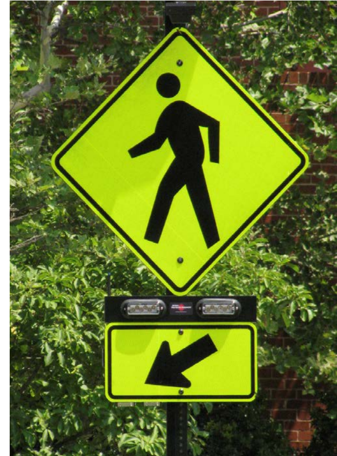
Close-up example of RRFB
