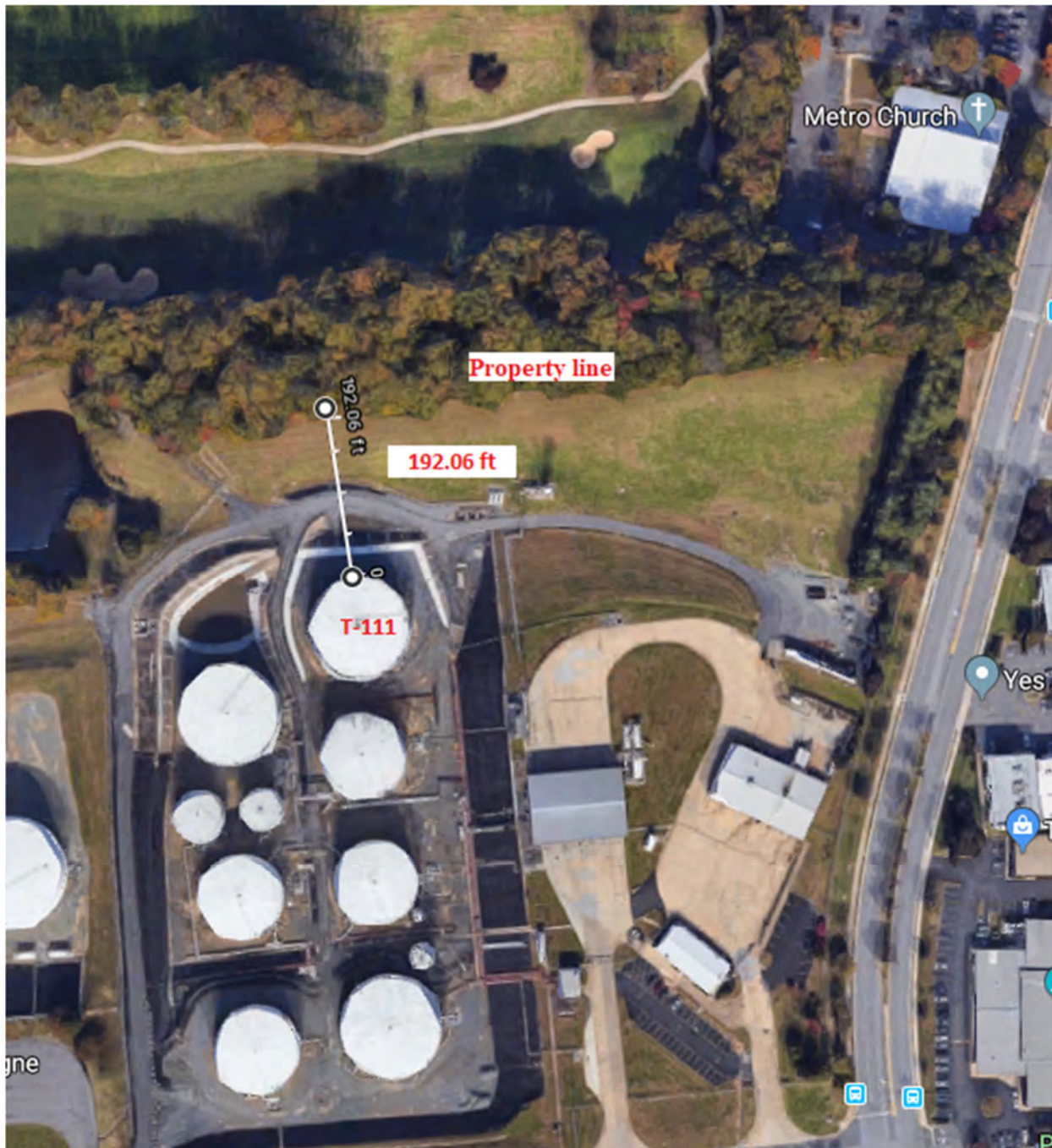
Figure 3 - Aerial view of the project site, showing actual distance between Tank T-111 and the property line is approx. 192 ft
