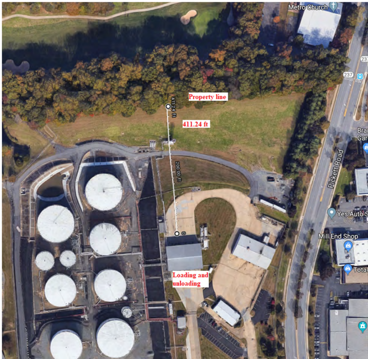
Figure 4 - Aerial view of the project site, showing actual distance between fuel loading / unloading area and the property line is approx. 411 ft
