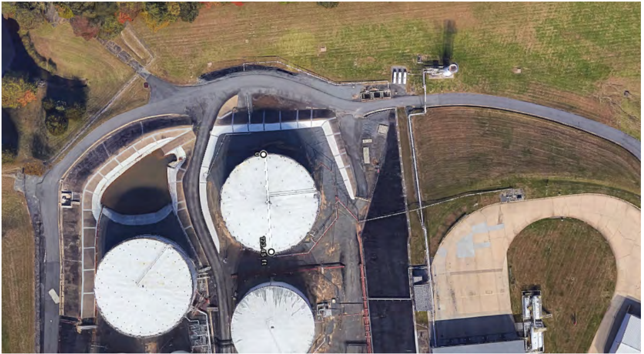
Figure 2 – Aerial view of Tank T-111, showing the tank diameter is approximately 124 ft.
