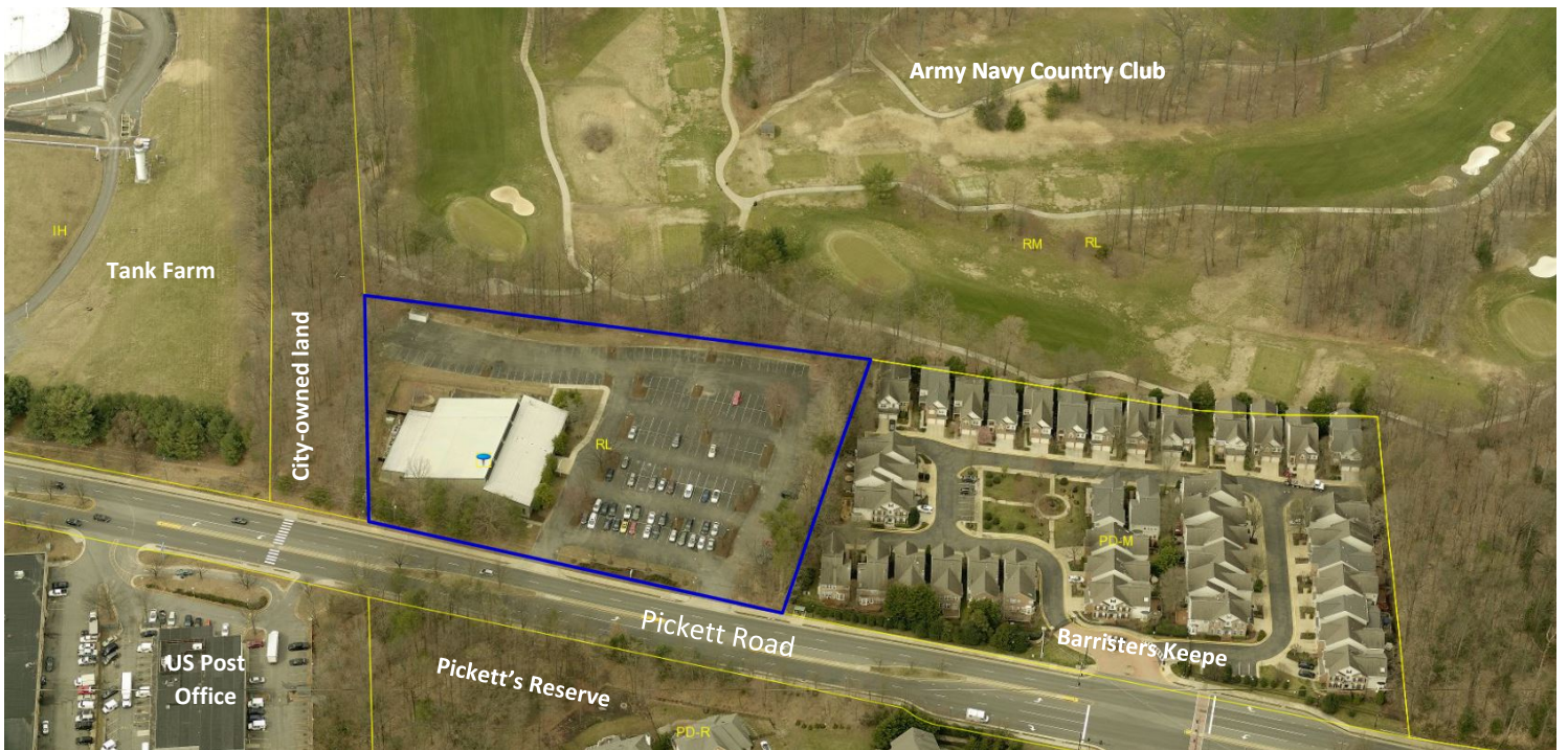
Aerial facing west
