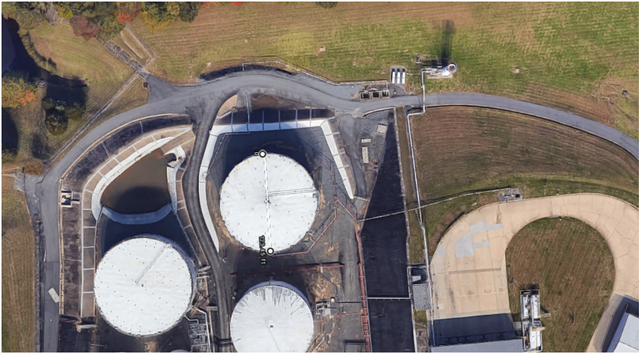
Figure 2 – Aerial view of Tank T-111, showing the tank diameter is approximately 124 ft.
