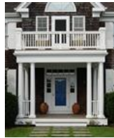
Jamestown Porch Railing
