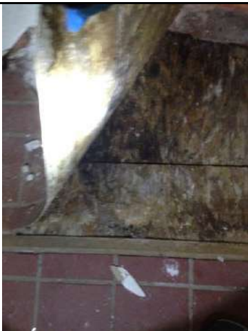
5. View of water impacts and mold beneath the sheet flooring in the laundry hallway.
