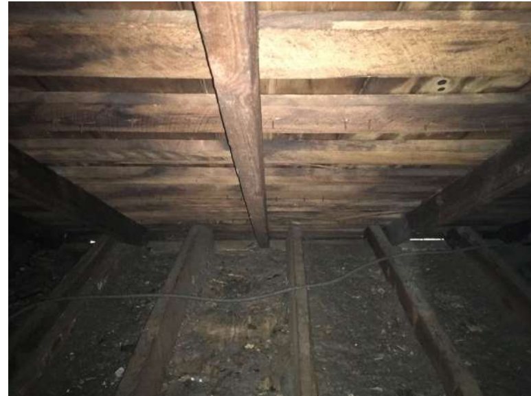
Typical roof rafter.
