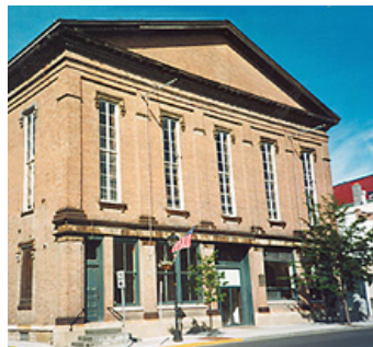
At the Hudson Opera House, a multi-arts center in Hudson, New York, the historic structure report was prepared incrementally. The first phase of the report focused on assessment and recommendations for repair of the roofing, the most critical issue in preservation of the building. Photo: Gary Schiro.
