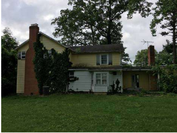
Flat roof at garage and laundry area
