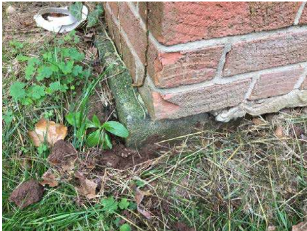
Rear chimney bottom
