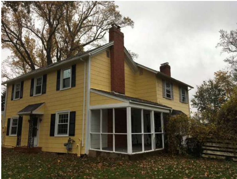
Southeast corner of building.
