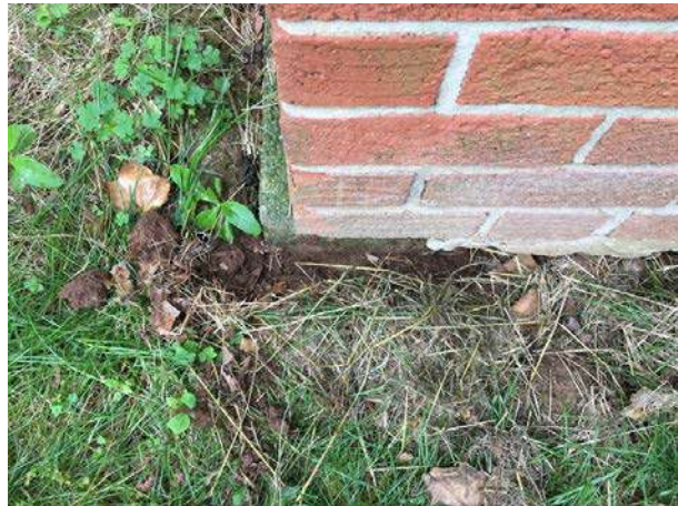
Rear chimney bottom
