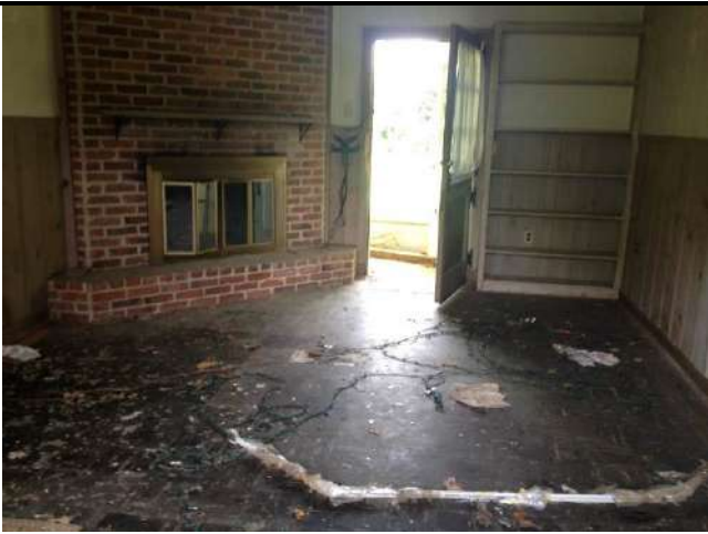
1. View of the den with 9" x 9" black floor tiles (ACM), Samples 1-2.
