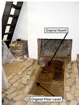
Archeological studies may be valuable in uncovering important evidence of changes to a historic structure. Following historical research and after several archeological soil probes, a decision was made to excavate an area in front of a mid-nineteenth century fireplace, revealing the original dirt floor and hearth undetected by earlier restoration efforts. Photo: NPS files.
