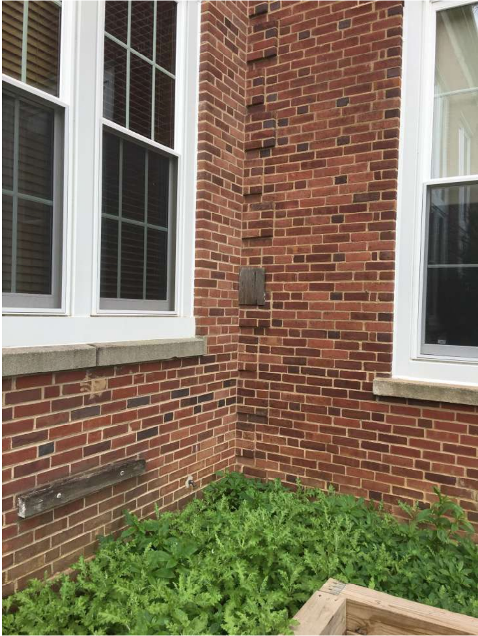
Photo #6: Front elevation at building corner
