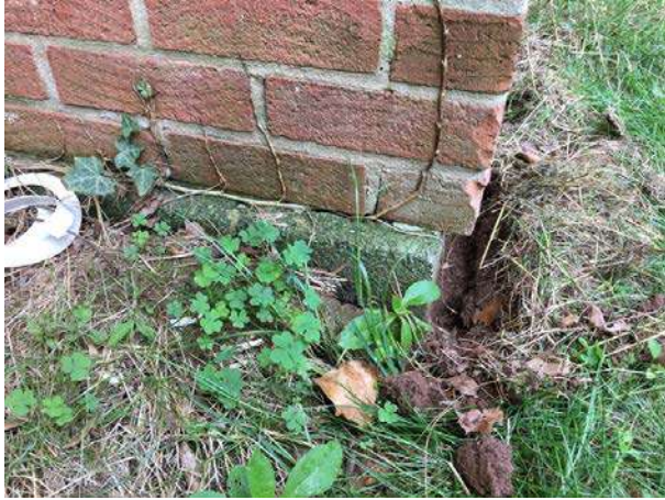
Rear chimney bottom
