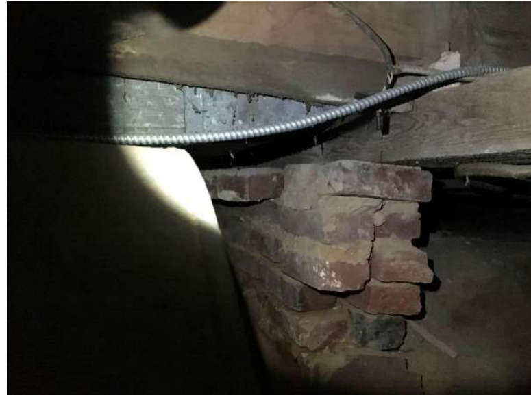
Partially collapsed masonry foundation.
