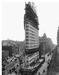
Historical research is directed toward gathering information on a structure's history, original construction and later modifications, occupancies, and uses over time. Research may range from national repositories such as the Library of Congress to local collections or private family records. Old newspapers, architectural journals and even manufacturing trade catalogs can be surprising sources of historical accounts and illustrations. This circa 1902 photograph of New York's Flatiron Building is of the construction in progress; such photographs are useful in understanding building chronology as well as concealed conditions of as-built construction such as building framing. Photo: Library of Congress, LC-D401-14278.
