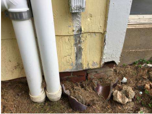
Downspout damaged
