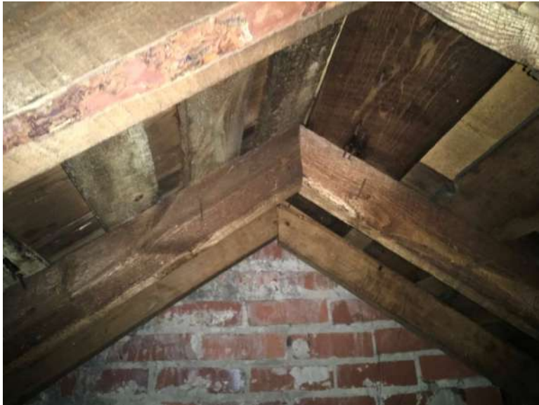
Typical main building gable roof framing.
