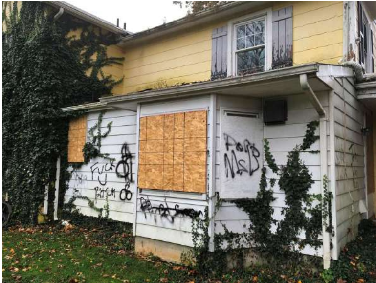
North elevation of property.
