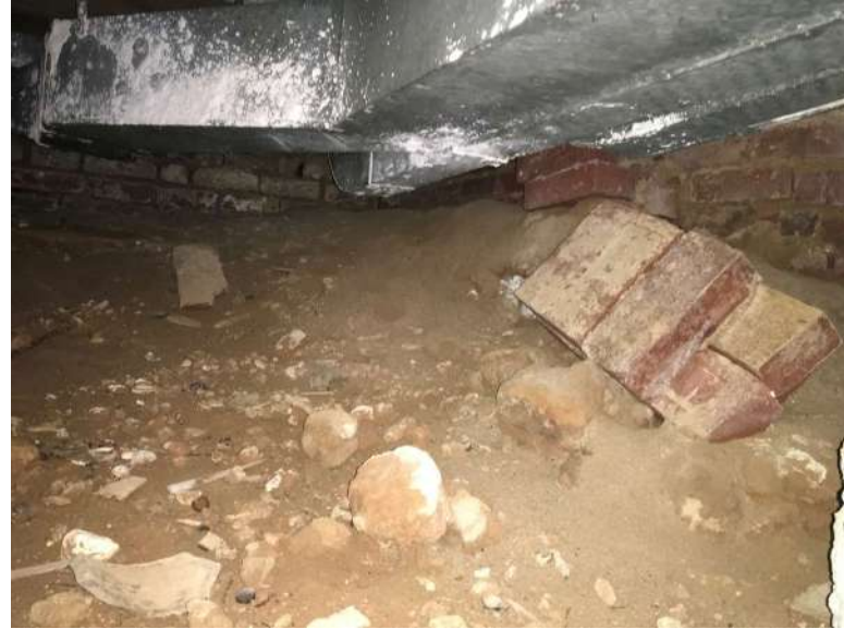
Partially collapsed masonry foundation.
