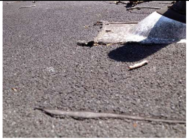
20. View of the black seam sealant (ACM), Samples 63-64.
