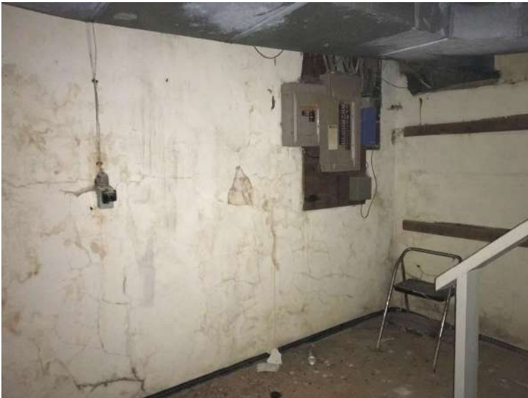
Cellar level under structure.
