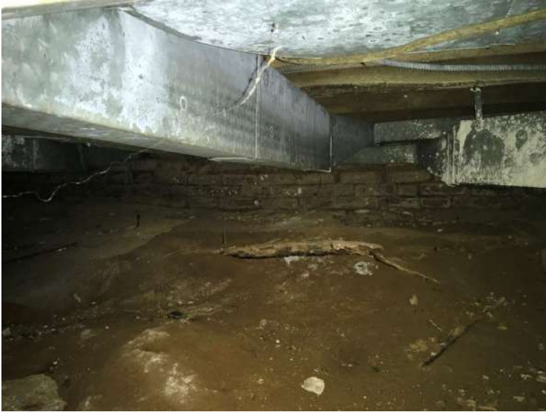
Crawl space under main portion of structure.
