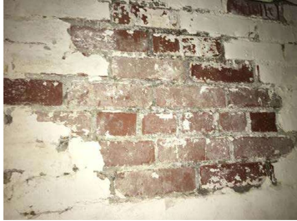
Exposed area of basement wall
