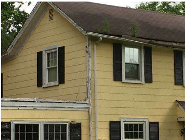
Typical roof condition
