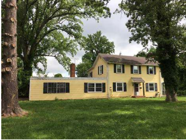
Gutters at the front
