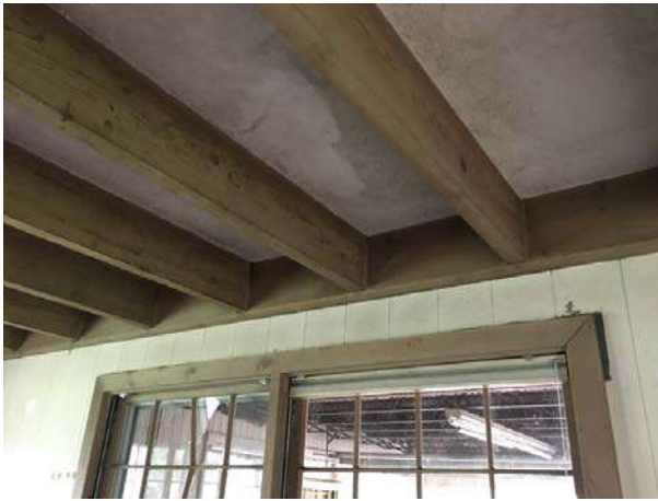
Exposed joists in room adjacent to garage
