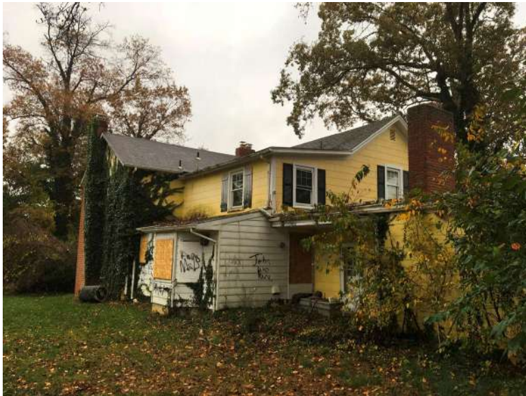
North elevation of property.
