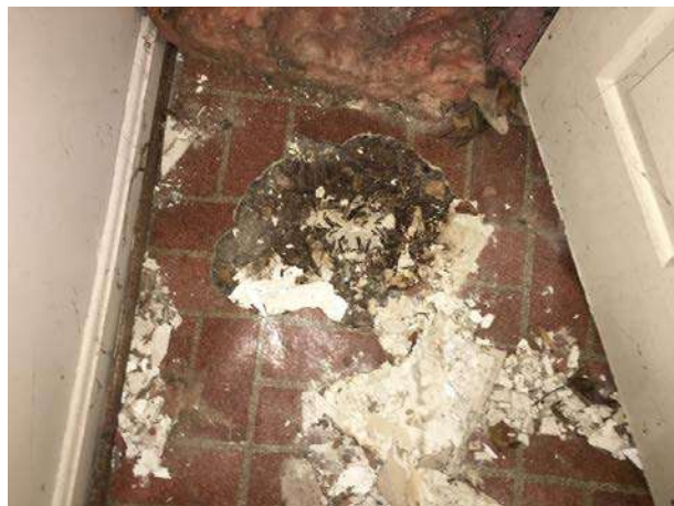
Flooring in the laundry room
