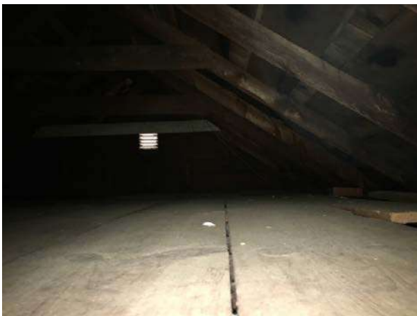
Rafter system supporting roof
