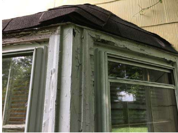
Shingles over bay window
