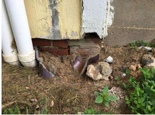
Downspout damaged
