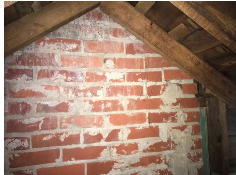
Brick wall at gable end.
