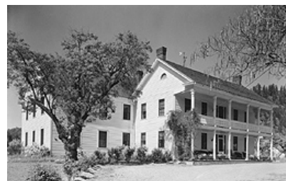
The treatment approach selected for a building usually is determined by the intended use of a property, funding prospects, and the findings of an investigation. The Wolf Creek Inn, operated by the Oregon Parks and Recreation Department, is among the most intact and oldest active traveler's inns in Oregon. The historic structure report outlined a rehabilitation treatment which included such work recommendations as repairs to specific historic fabric, landscape restoration and site improvements, and upgrading of the building's mechanical and electrical systems. Photo: Historic American Building Survey, 1934.
