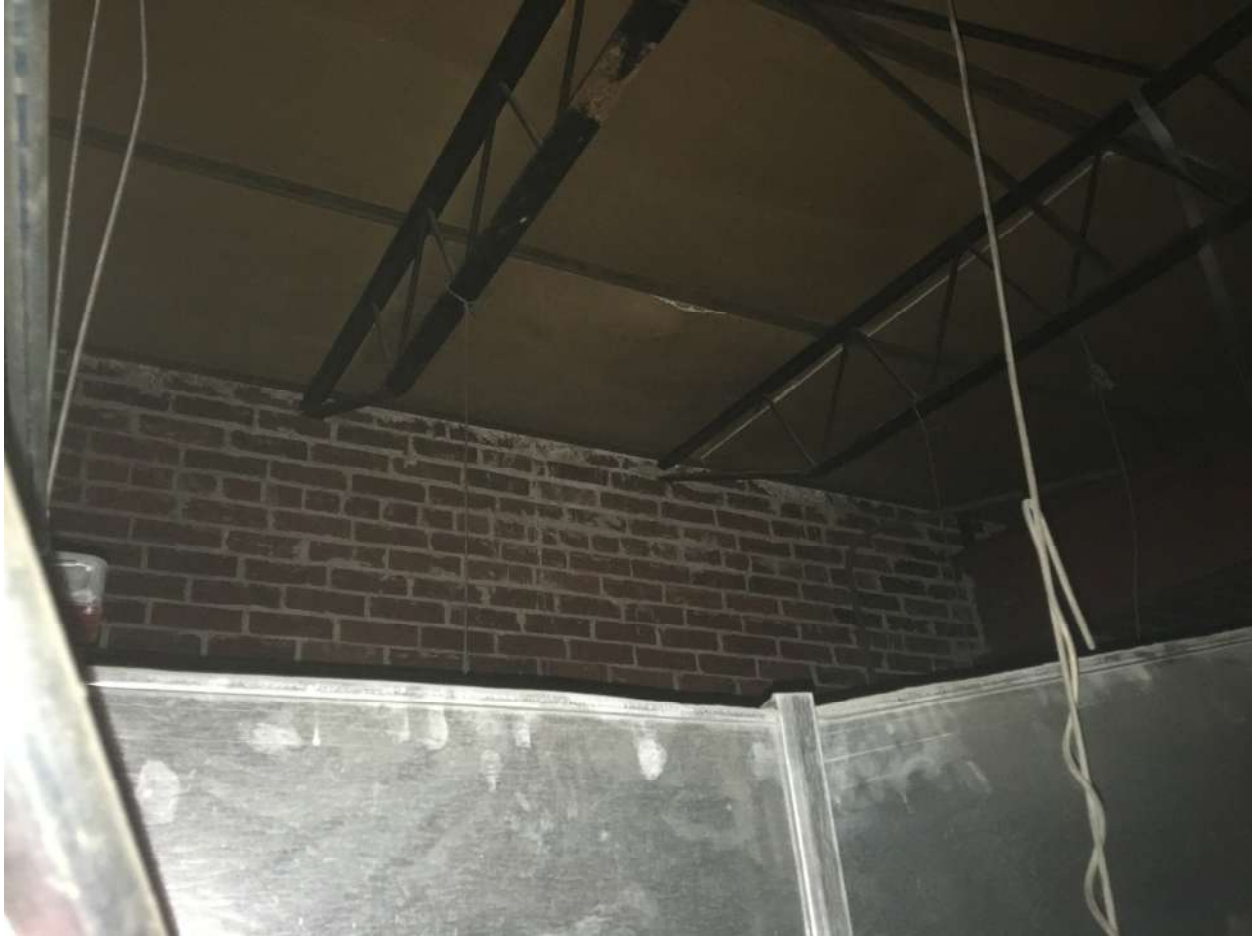
Photo #3: Roof joist bearing on interior brick wall.
