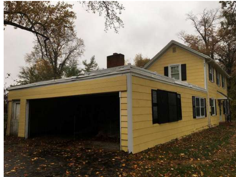
West side of building.
