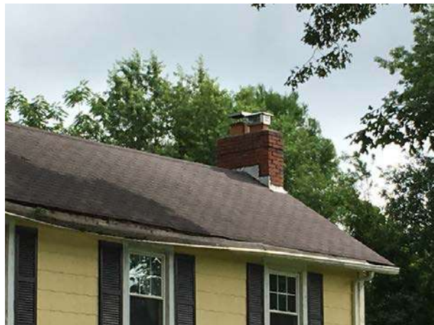
Typical roof condition
