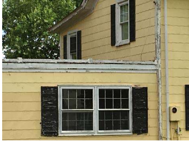
damaged gutters
