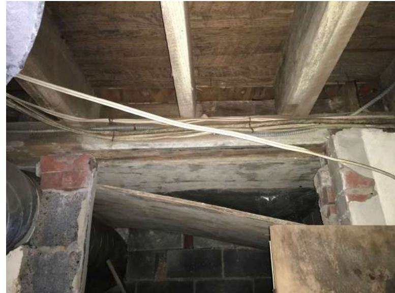
Floor support beam spanning opening.
