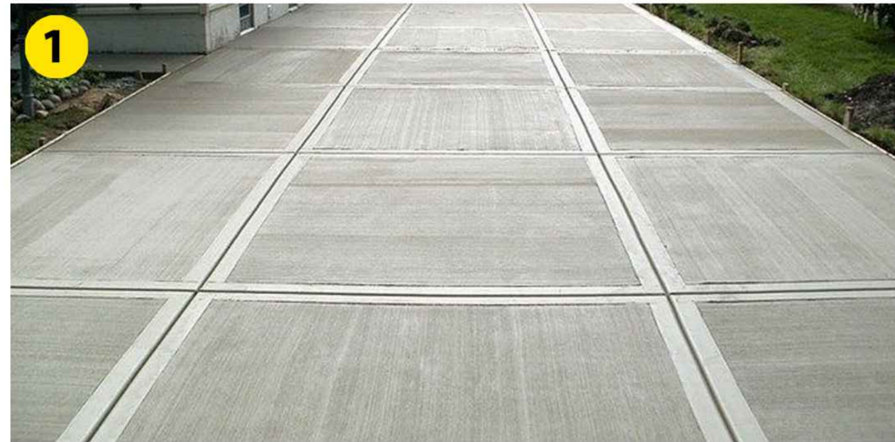
BRICK EDGING AT CONCRETE
