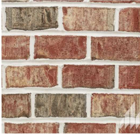
BRICK VENEER SPALDING TUDOR
