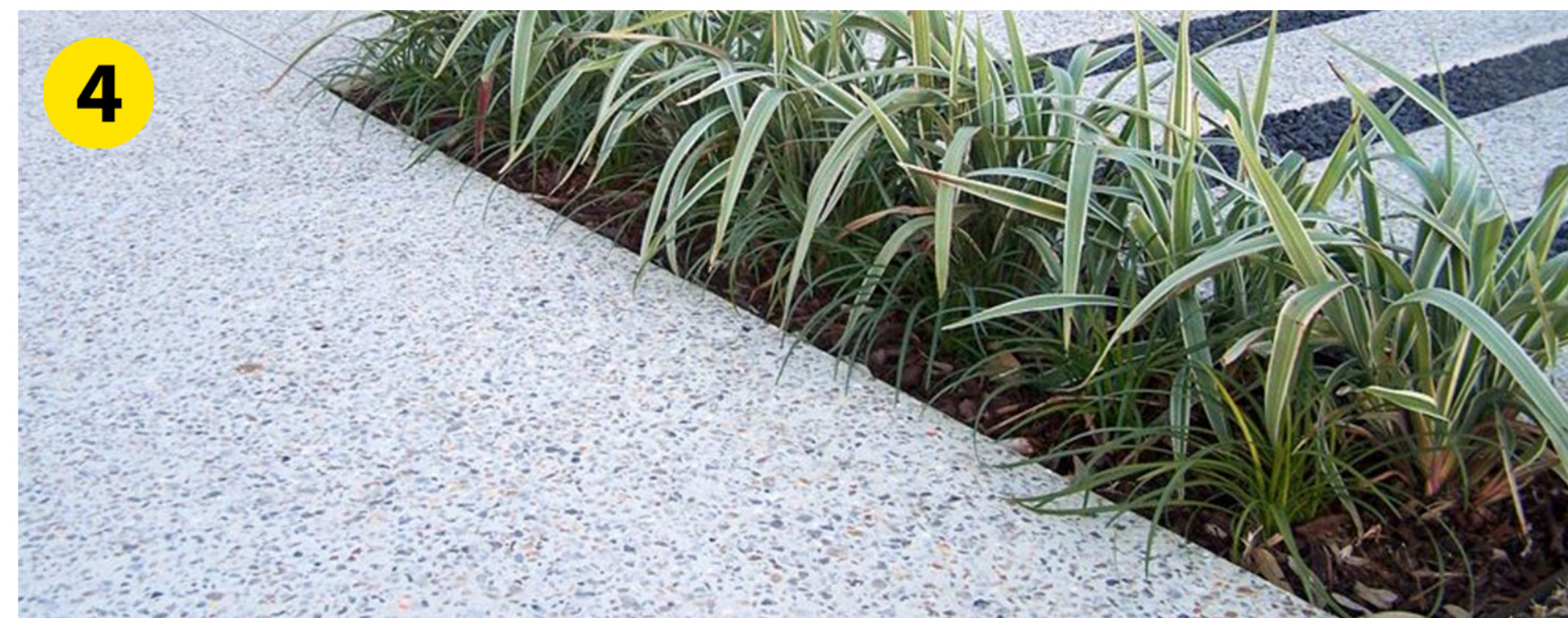
EXPOSED AGGREGATE CONCRETE PATHWAY AT CEDAR AVENUE
