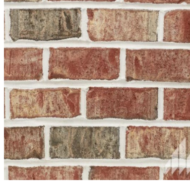
BRICK VENEER SPALDING TUDOR
