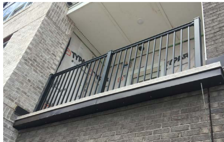
Photo Example of the Black Metal Rails
