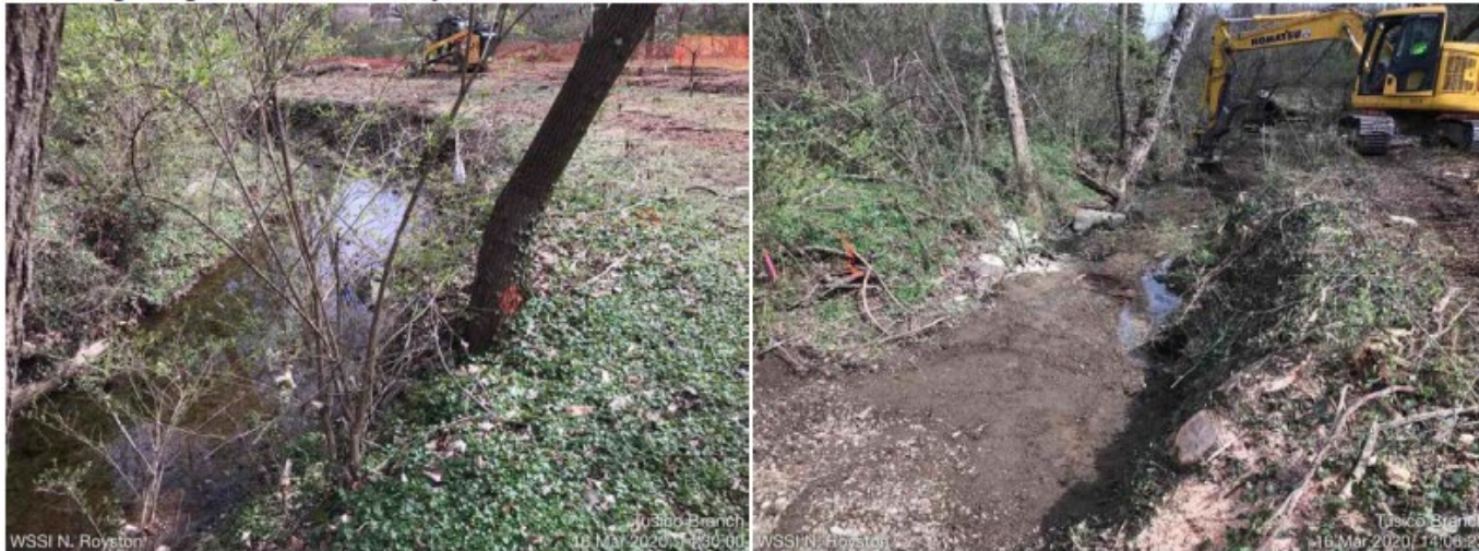
At the beginning of construction and just after tree removal, March 2020
