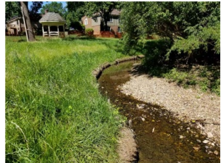
After Construction & Stabilization, June 2020
