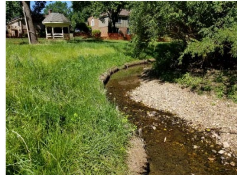
After Construction & Stabilization, June 2020
