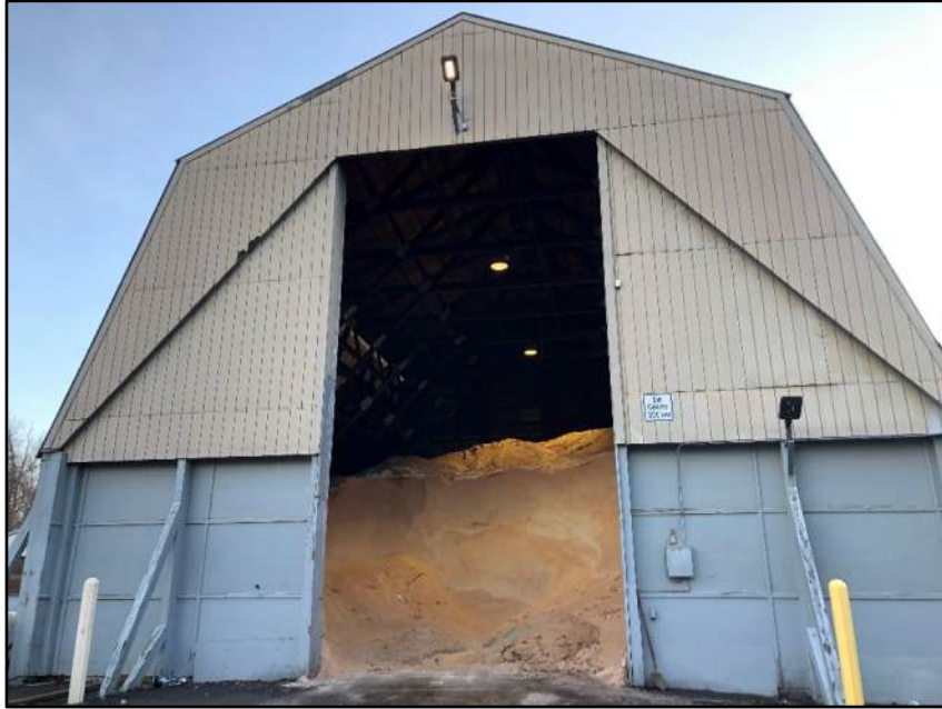
Figure 4. Covered on-site salt storage (2021)
