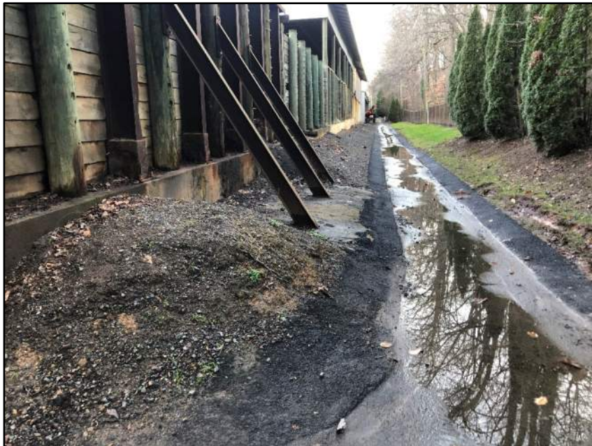
Figure 5. On-site swale in proximity to aggregate/salt storage (2021)
