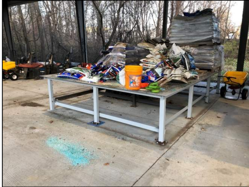
Figure 6. De-icing chemicals elevated above floodplain (2021)
