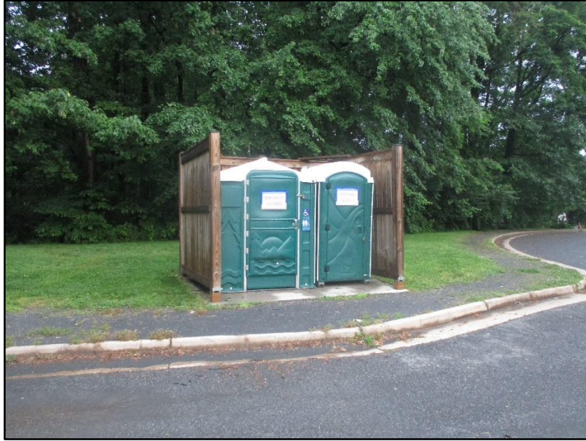
Figure 4. On-site portable sanitation facilities.
