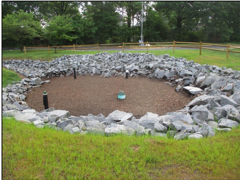
Figure 11. On-Site Bioretention Facility
