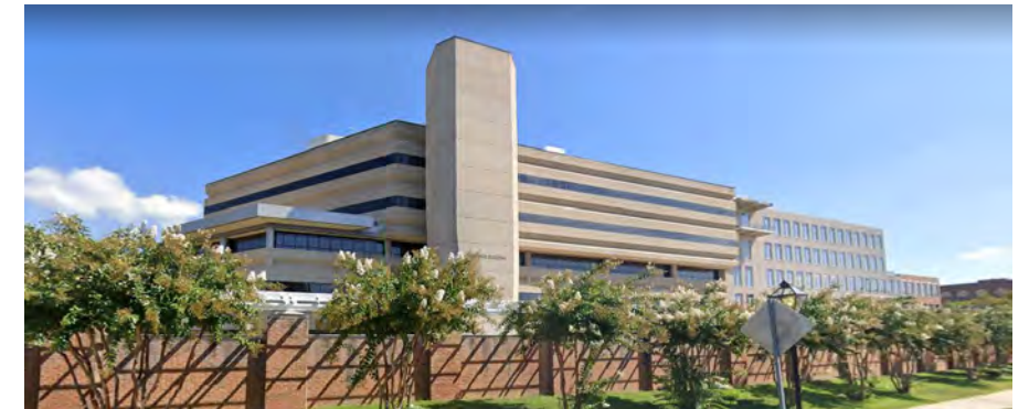
3 FAIRFAX COUNTY DETENTION CENTER
