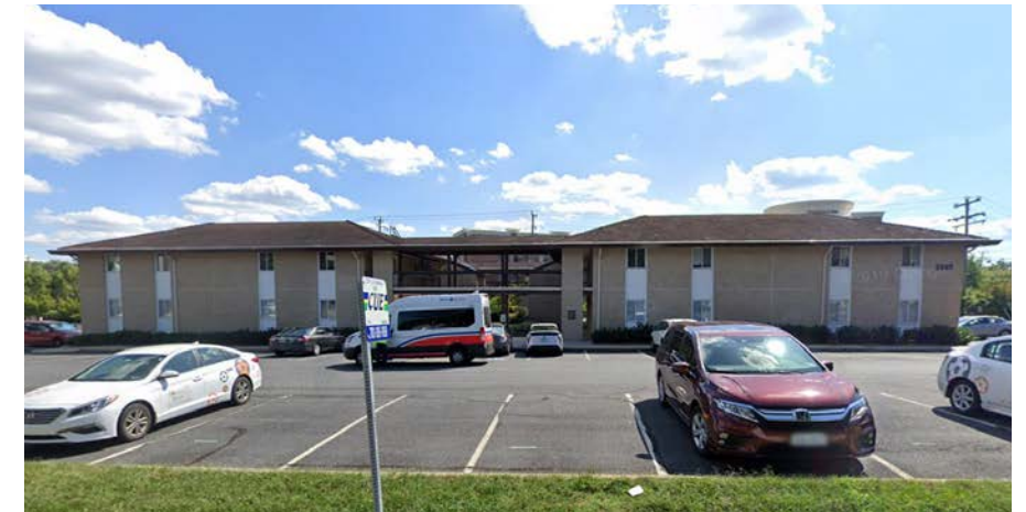
② 3541 CHAIN BRIDGE RD, FAIRFAX, VA 22030
