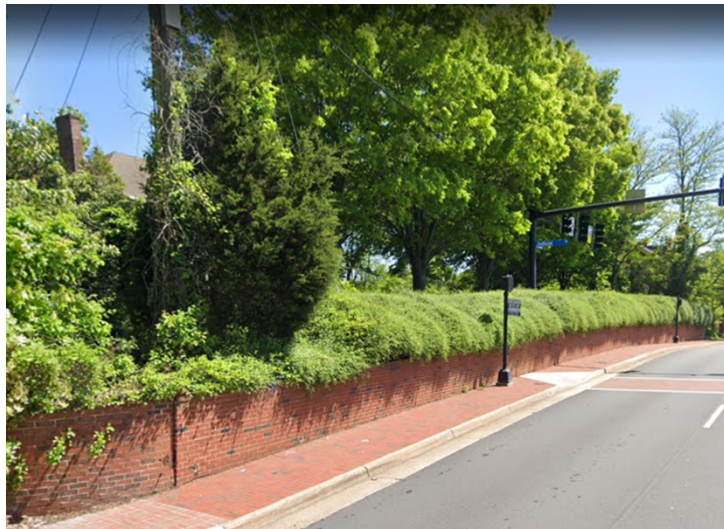
View Along Chain Bridge Road
