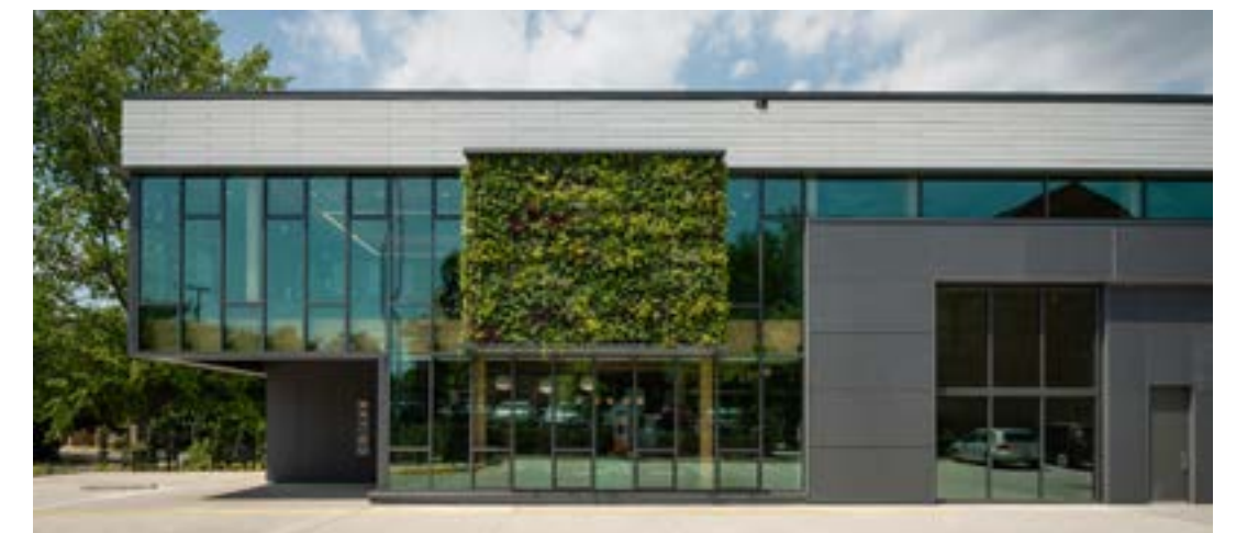
HITT Construction CoLab (Image credit: HITT Contracting)
