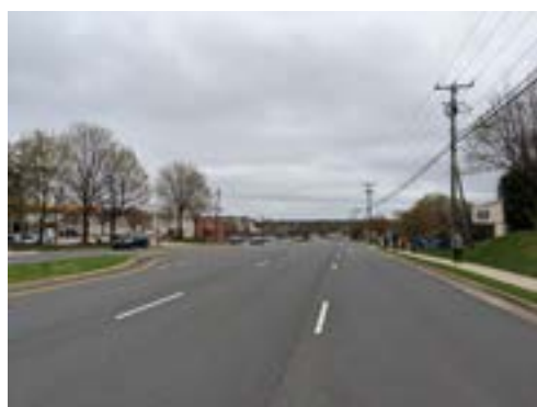
NARROW SIDEWALKS NEXT TO WIDE ROADS
