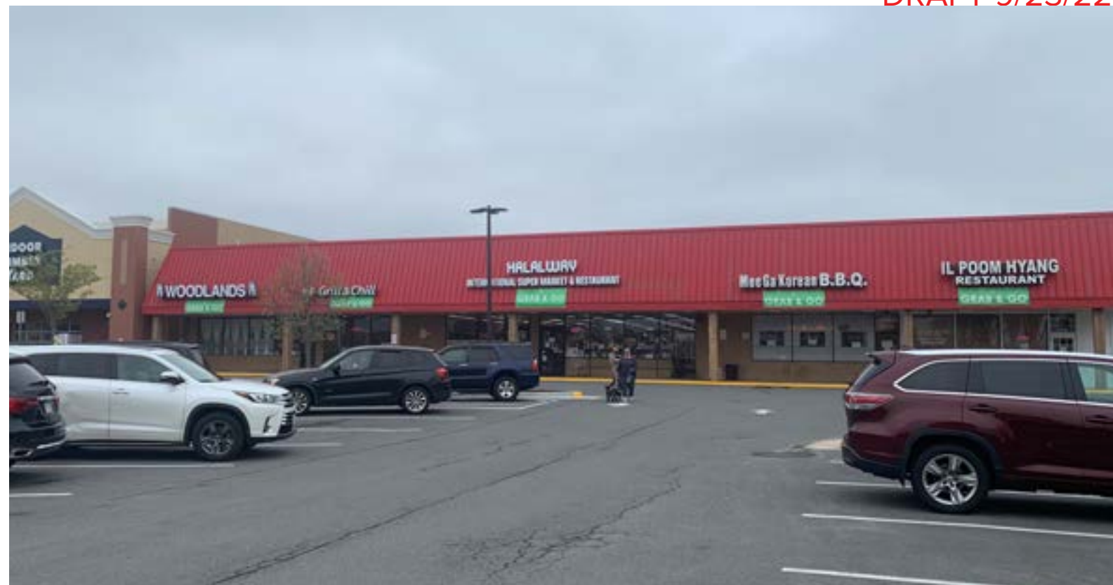
EXISTING CAR ORIENTED RETAIL FORMAT CURRENTLY TYPICAL TO KAMP WASHINGTON
