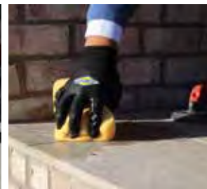
PIC 2. Remove excess grout with clean water.
