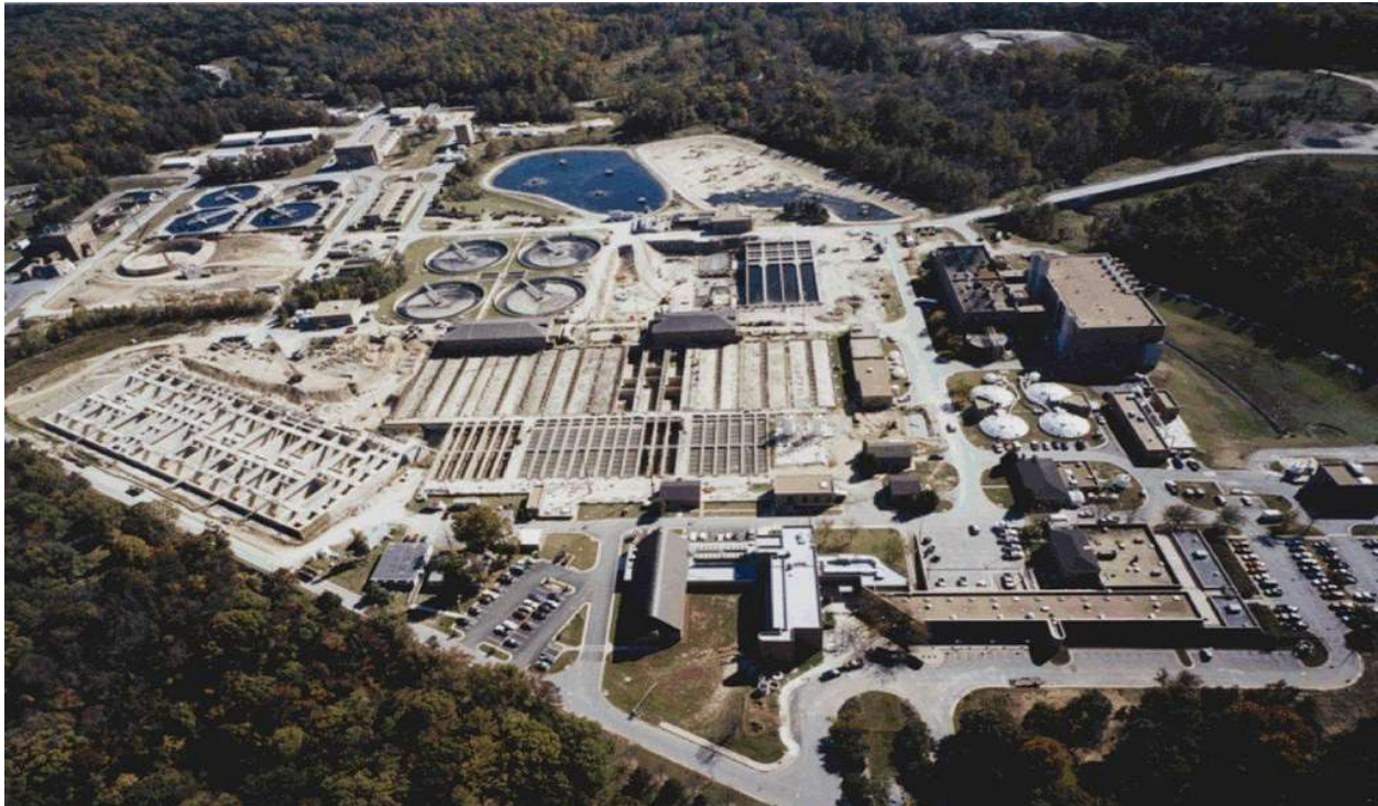
Noman M. Cole Wastewater Treatment Plant (Fairfax County facility where the City's wastewater is treated)
