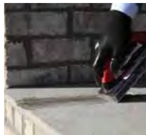
PIC 1. Fill joint with grout.
