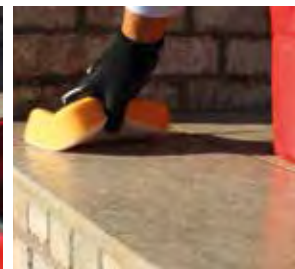
PIC 5. Removal of excess grout residues with hard brush.
