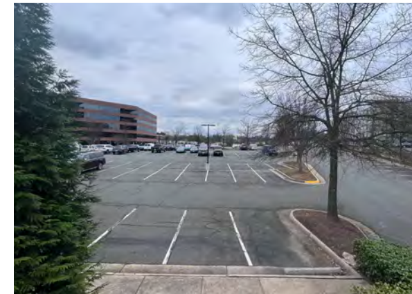
E VIEW LOOKING SOUTH FROM ADJACENT EXISTING PARKING GARAGE
