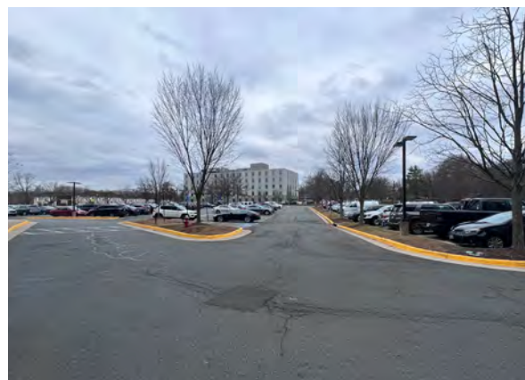
G VIEW LOOKING SOUTH WEST FROM ADJACENT OFFICE BUILDING
