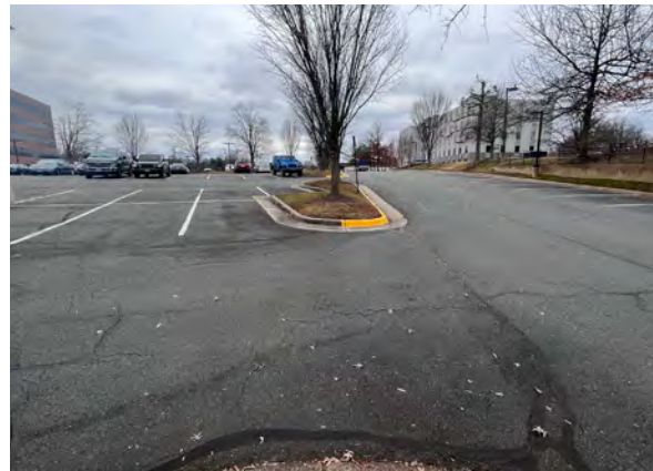
D VIEW LOOKING SOUTH EAST FROM EXISTING PARKING GARAGE ADJACENT ENTRANCE
