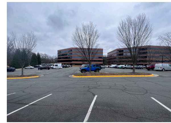
(C) VIEW LOOKING EAST FROM SITE INTERIOR
