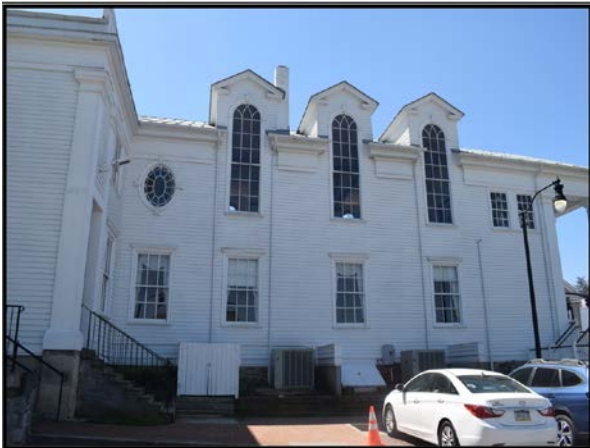
View of Old Town Hall from northern parking lot, facing south.
