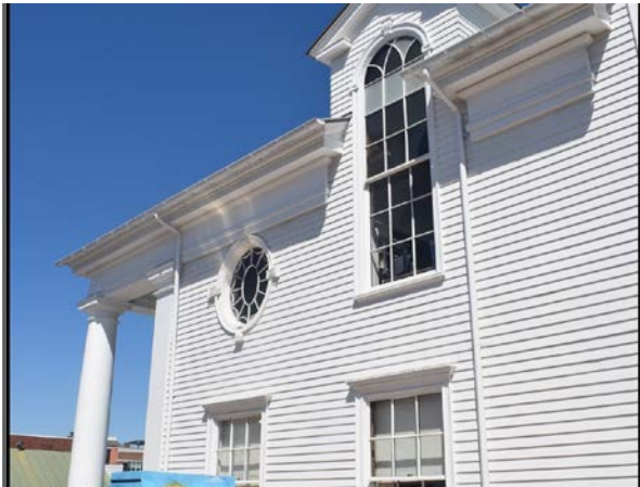
View of Old Town Hall south side, facing northwest.
