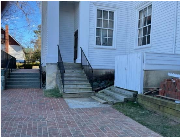
View of Old Town Hall northeast side stairs to be replaced.
