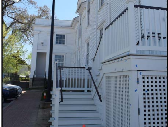
View of Old Town Hall northwest side stairs, facing east.
