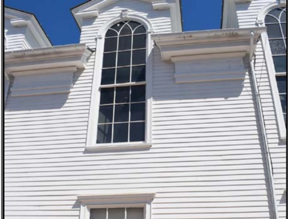
View of Old Town Hall south side, facing north.
