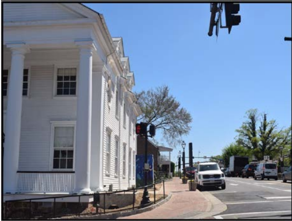
View of Old Town Hall west and south sides, facing east down Main Street.
