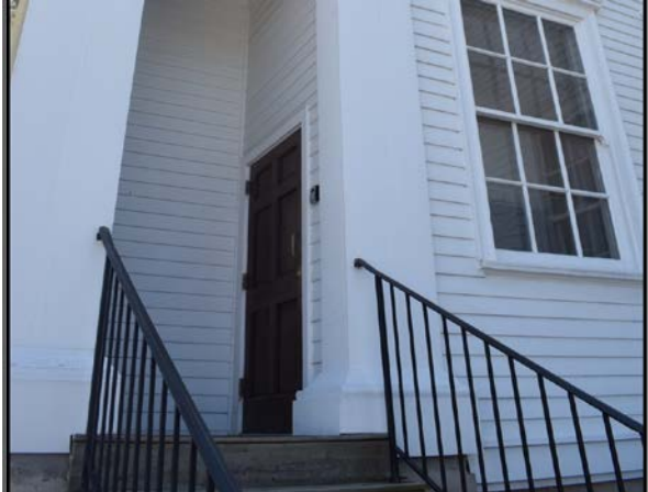
View of Old Town Hall northeast entry, facing southeast.
