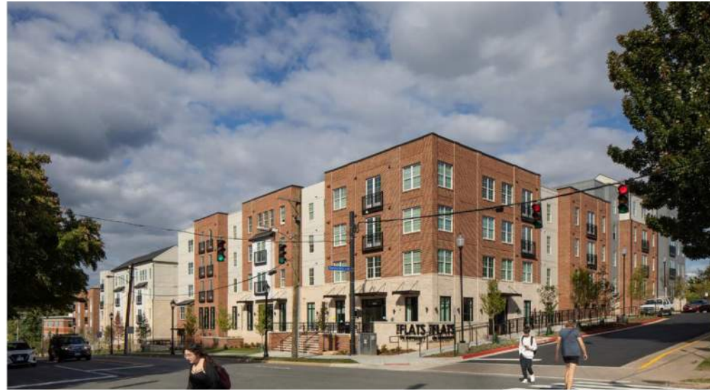
4085 CHAIN BRIDGE ROAD
