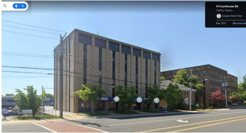
4085 CHAIN BRIDGE ROAD
