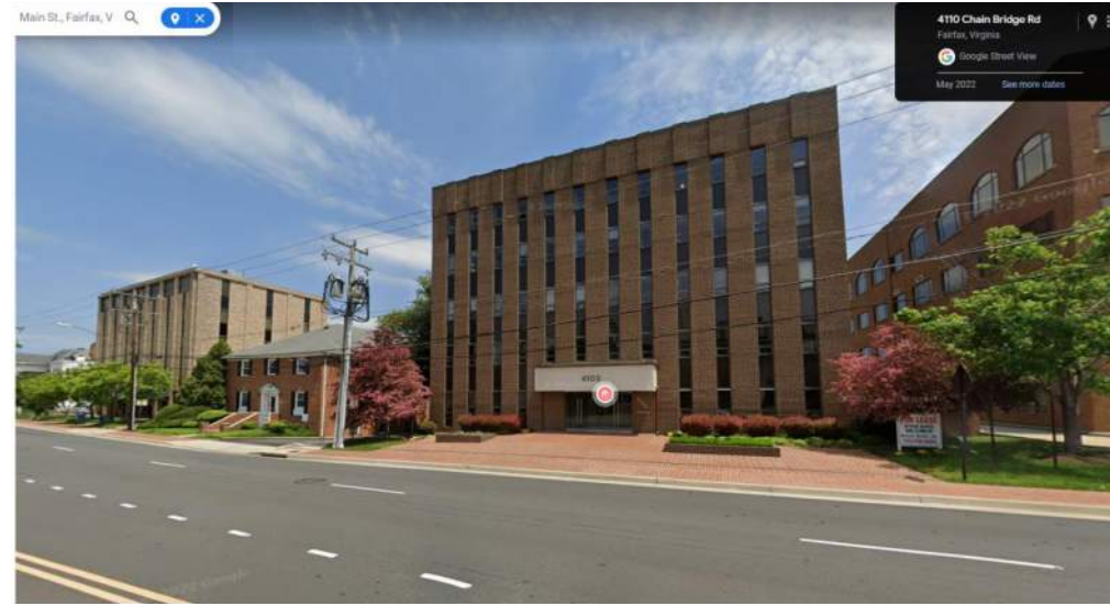
4103 CHAIN BRIDGE ROAD
