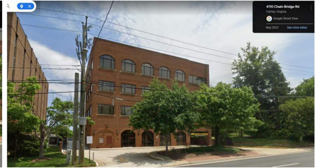
4117 CHAIN BRIDGE ROAD
