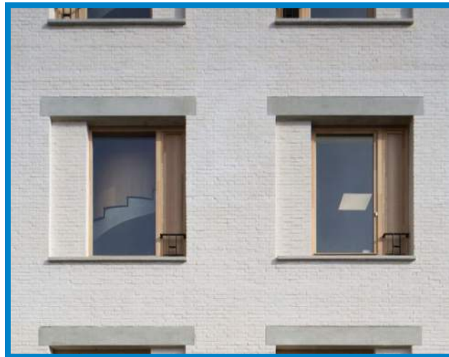
4 PAINTED ARCHITECTURAL LINTEL / HEADER
