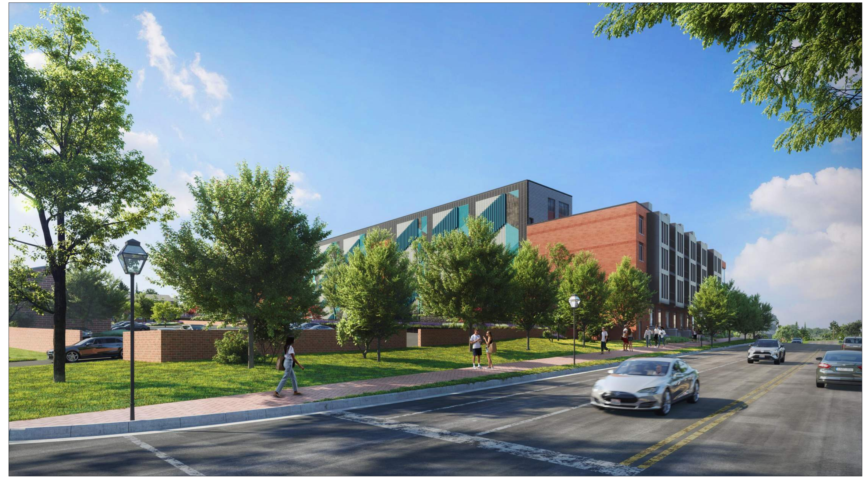
② UNIVERSITY DR VIEW LOOKING NORTHWEST
