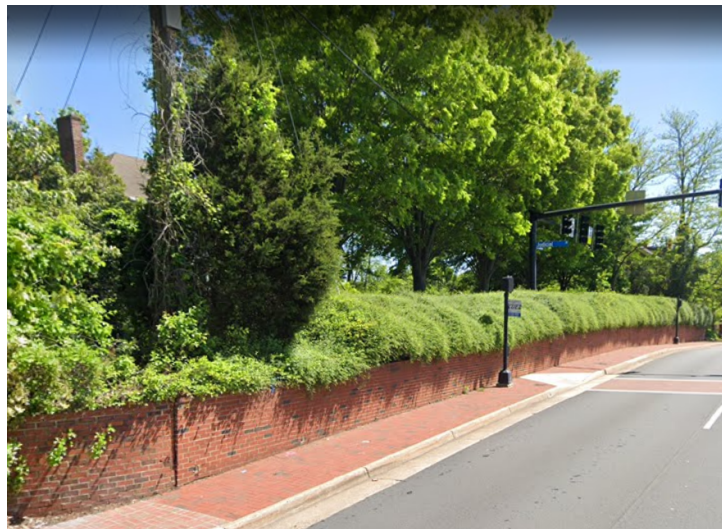
View Along Chain Bridge Road
