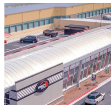
R-1 ROOF SYSTEM ACRYLIC ROOF PANELS FOR ILLUSTRATION OF ROOF MATERIAL ONLY
