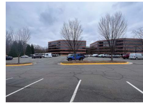
(C) VIEW LOOKING EAST FROM SITE INTERIOR
