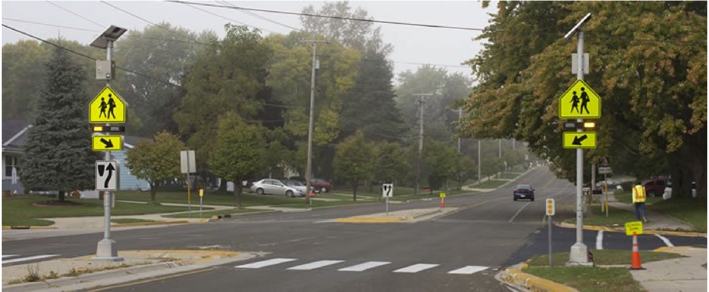
Rectangular Rapid Flashing Beacon (RRFB)
