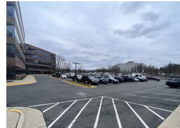
F VIEW LOOKING SOUTH FROM NORTH EAST SITE CORNER
