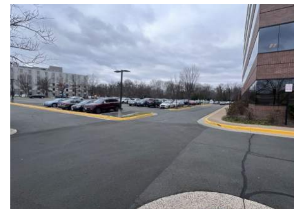
I VIEW LOOKING NORTH FROM EAST SITE ENTRANCE
