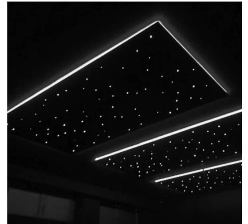
PINHOLE STARLIGHTS LOCATION: MAIN ENTRANCE SOFFIT
