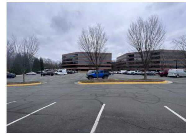
C VIEW LOOKING EAST FROM SITE INTERIOR
