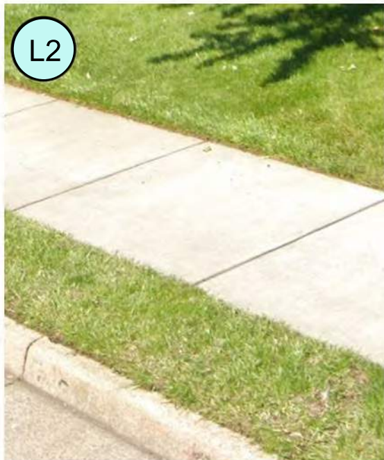
Concrete Paving: Cast in Place
